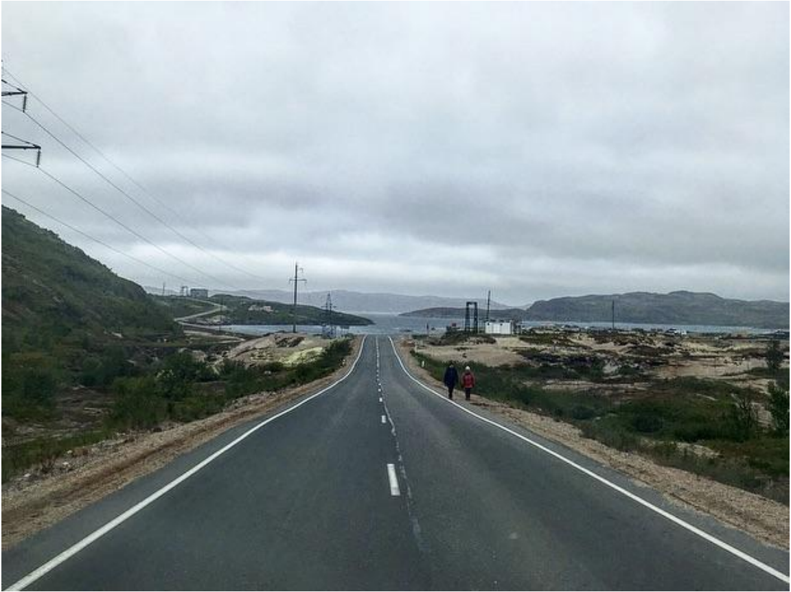
Figure 15. The asphalted road within the Teriberka village. July 12, 2019.
