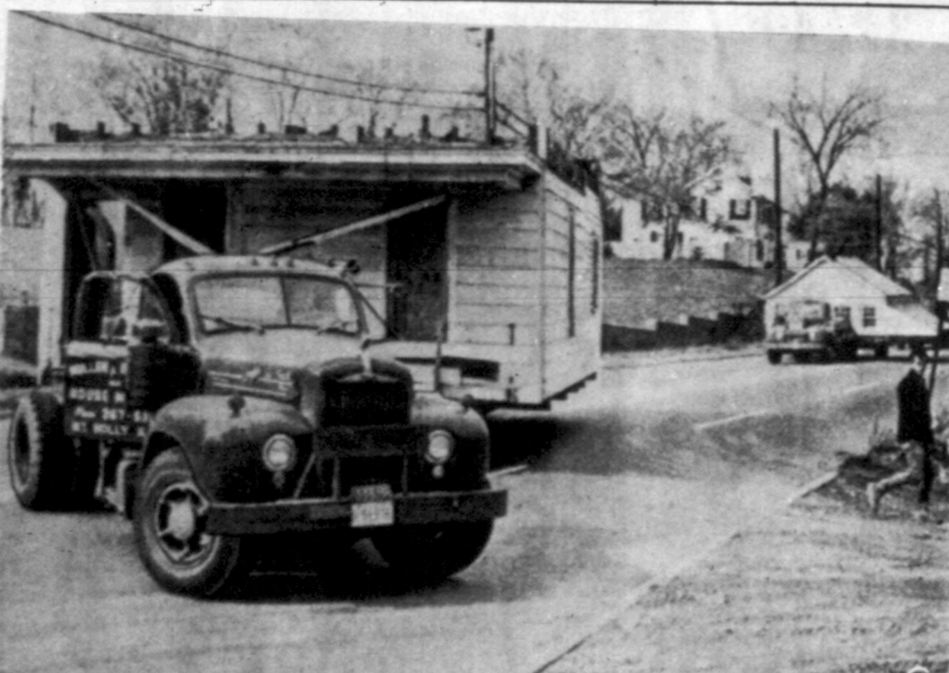
A DIVIDED HOUSE —This 200-year-old "salt box" house was sawed in half before being moved on two trailer trucks to Speedwell Historical Village in Morristown, N.J., for re-assembly. The first floor is on the front truck.
