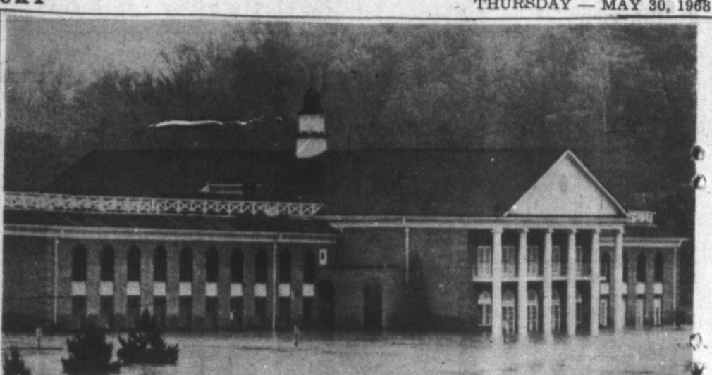
COLLEGE CAMPUS FLOODED IN SOUTHERN OHIO—The worst floods in southern Ohio since the 1913 "holocaust by water" covered the Ohio University campus in Athens knee-deep.
