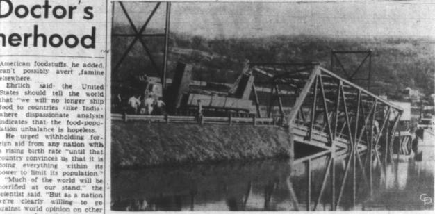
NO CLEARANCE A bridge collapse where Short Creek flows into the Ohio River at Warrenton, Ohio, finds one tractor trailer in the middle and one that just missed. The load on the trailer in the middle struck the bridge's top and down it went.
