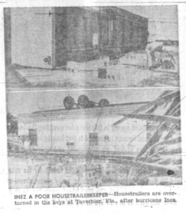
INEZ A POOR HOUSETRAILERKEEPER—House trailers are overturned in the keys at Tavernier, Fla., after hurricane Inez.
