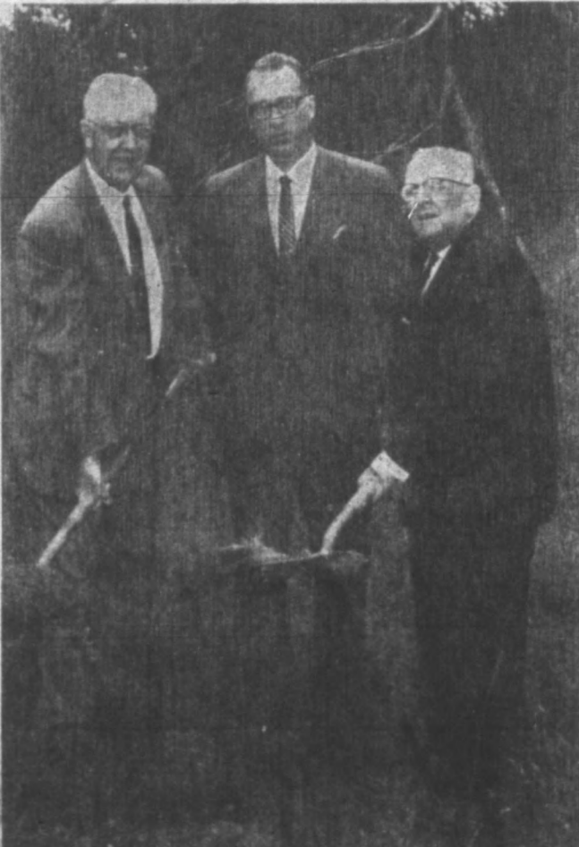
Dr. Ralph H. Woods, left and George Hart, right, break ground for the new Bob White Dormitory which will house 400 students. In the center is Blair Wright, general contractor of Memphis, Tennessee. This dormitory will be located on the south side of Chestnut street just west of Bailey Pump and Pipe Company and is the first in a complex of four dormitories.
