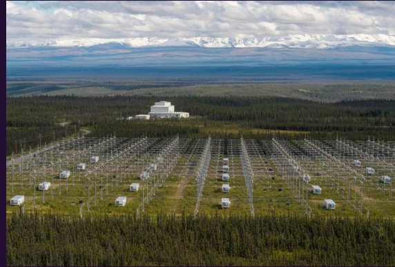
The HAARP facility as of September 5 th , 2018.
