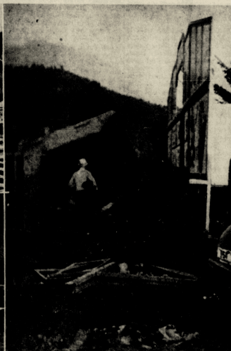
DAMAGE OF $20,000 was wrought by the flood to the J. F. Sparks carnival, part of whose wreckage is shown here. More than 150 employees of the carnival saved themselves by clinging to rooftops, trucks and trees.
