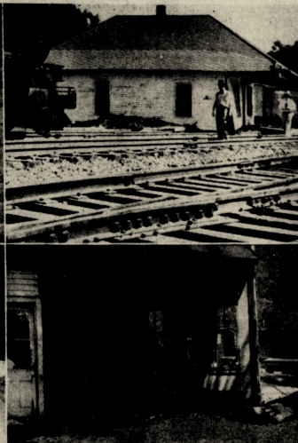
A HOUSE owned by Loren Fannin was washed (top) across the Chesapeake & Ohio Railway tracks, which themselves were damaged extensively. Below is the wreckage of a cleaning establishment which was washed off its foundations.
