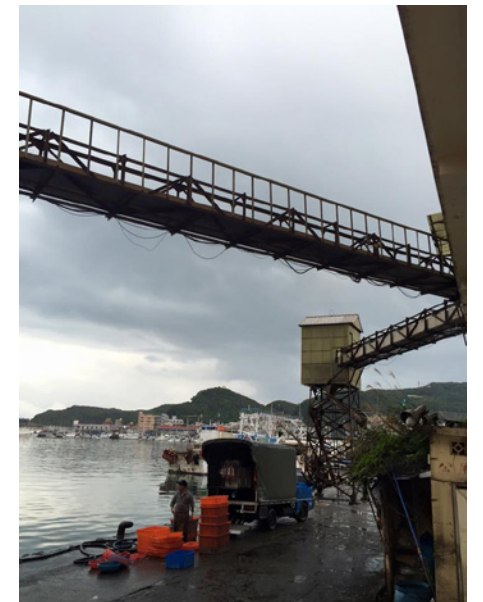
The ice blocks are transfer through a rail and can be crushed on demand.
