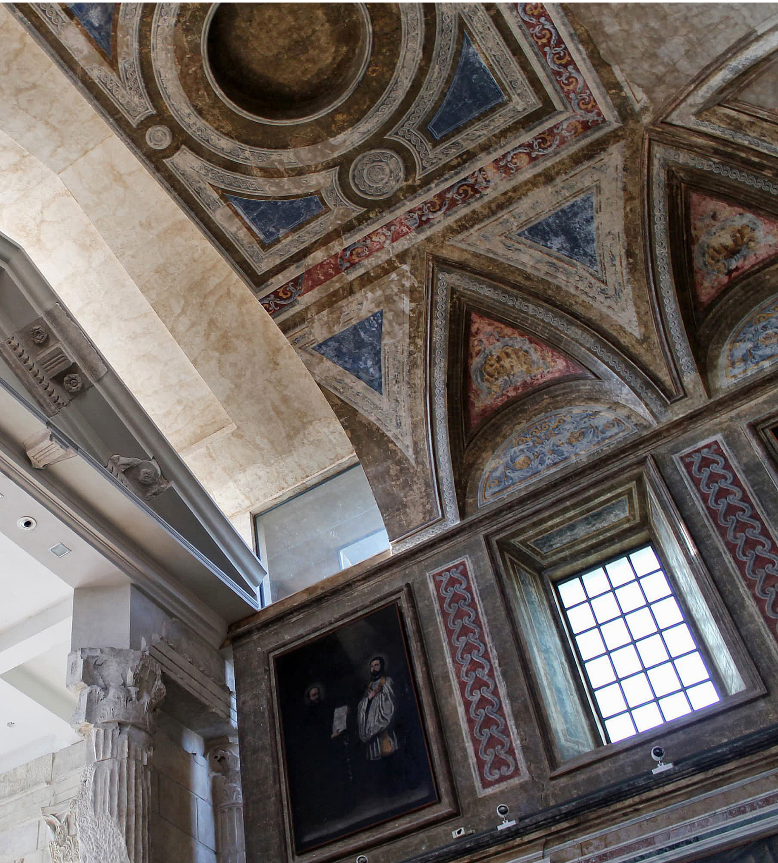
The gap between the reconstructed rear pediment of the temple and the lunette vault of the baroque chancel
