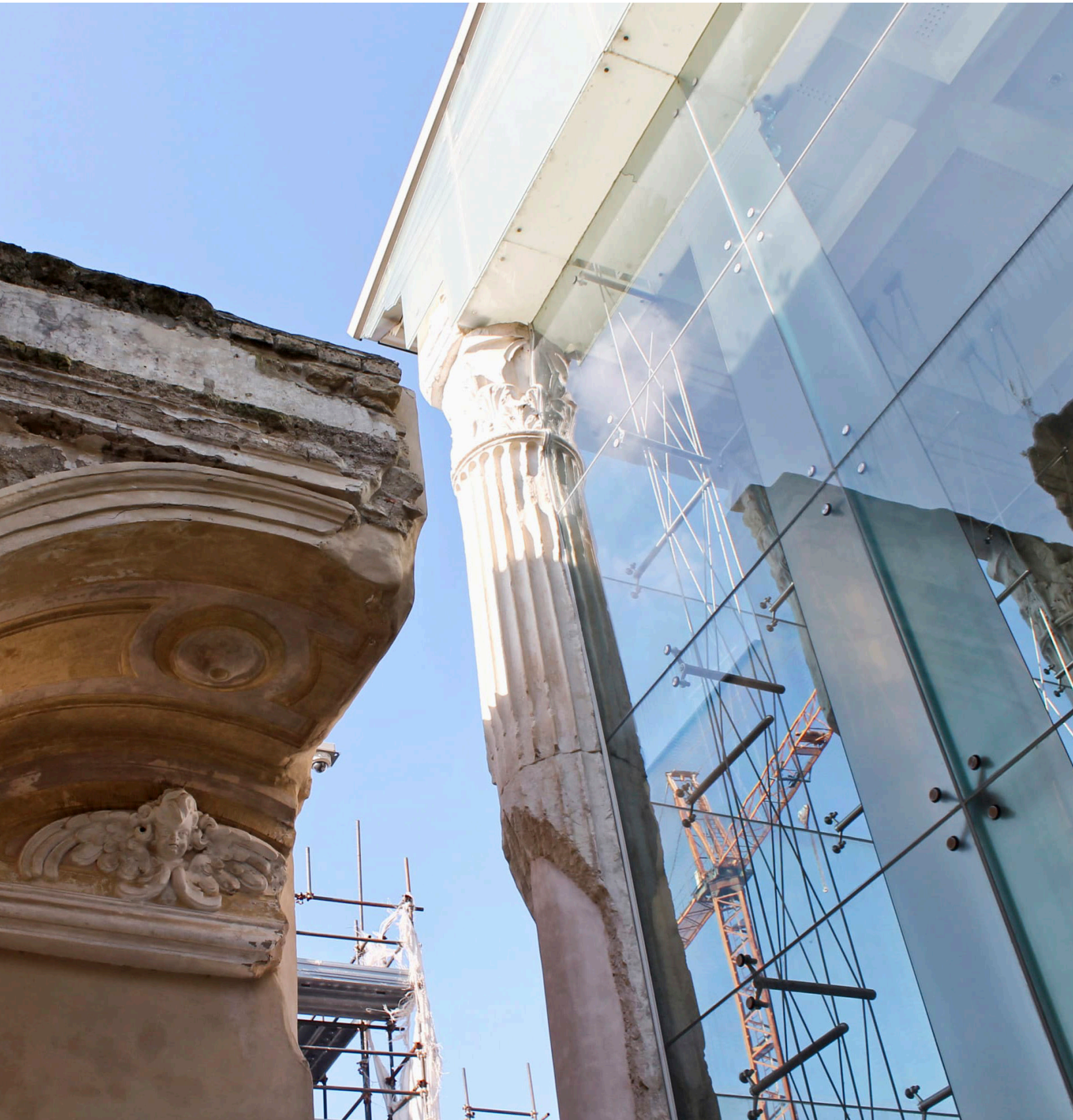
The remains of the first two lateral chapels of the XVII century and the angular columns of the pronaos of the temple, embedded in the new glass facade, delimit a kind of open vestibule to the cathedral
