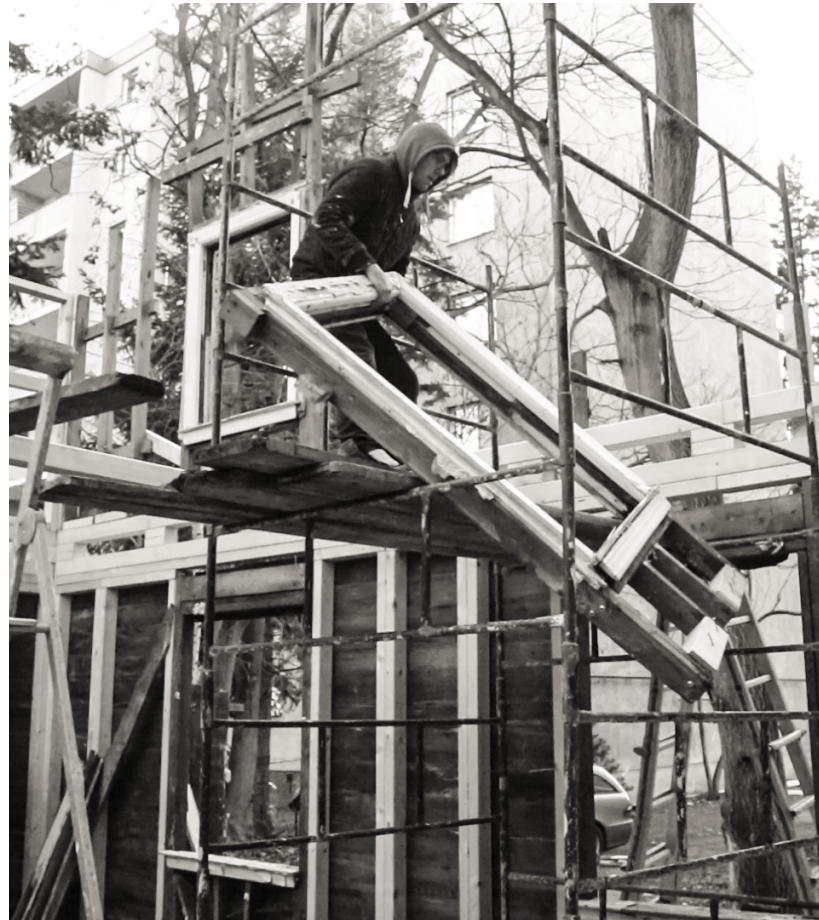
Ryan Mendoza reassembling the house in Berlin, Germany
