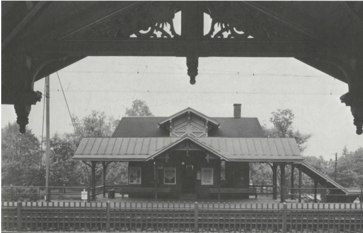
Platform Photograph of Inbound Station Building
