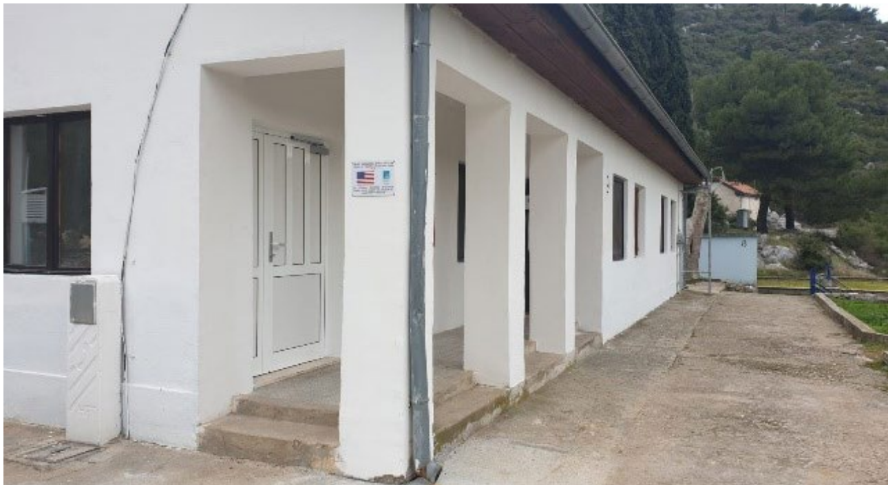
Entrance to warehouse Complex Tatinje
