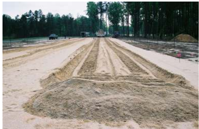
Figure A-12: Sifted Sand Lane with End-Berm
