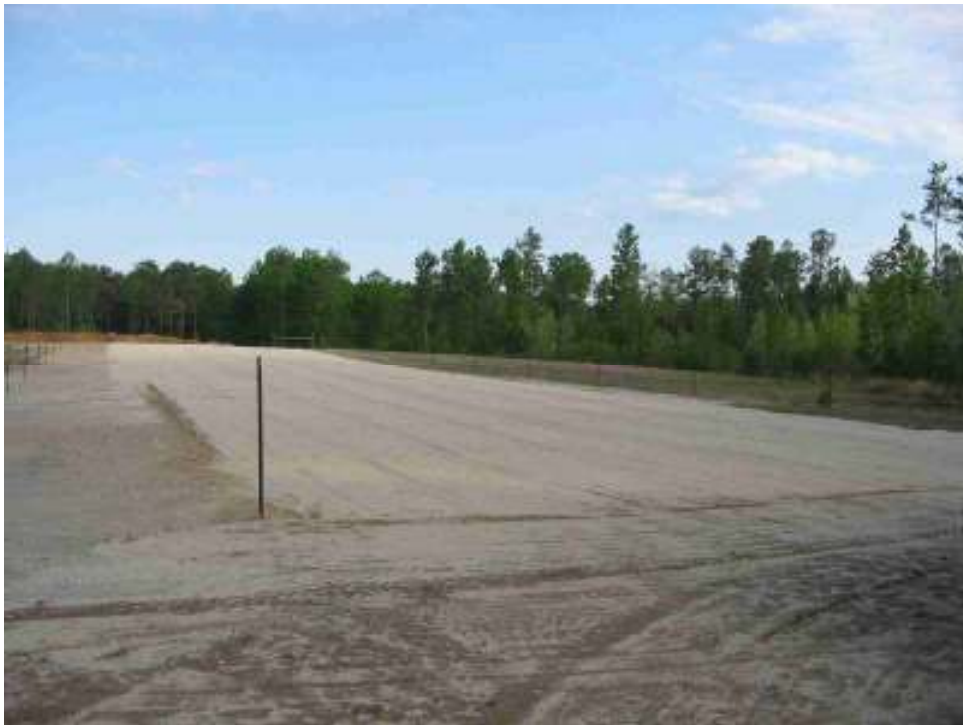
Figure 16: Test Site 3 – Sand
