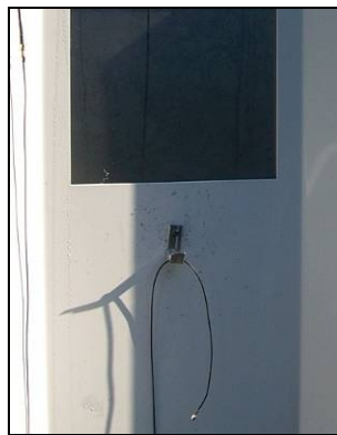
Figure 26: Remote Device Hook and Antenna Cable
