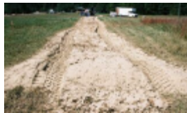
Picture 22 – Flailed lane
