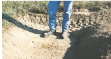
Picture 28 – Ditch dug by the flail
