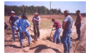
Picture 26 – Digging for the load cell in fluffy dust
