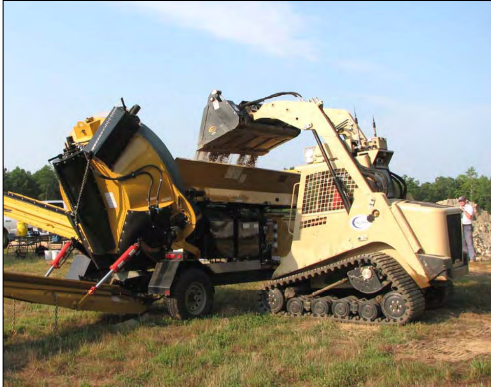
Figure 27: ASV SR-80 Loader in Operation
