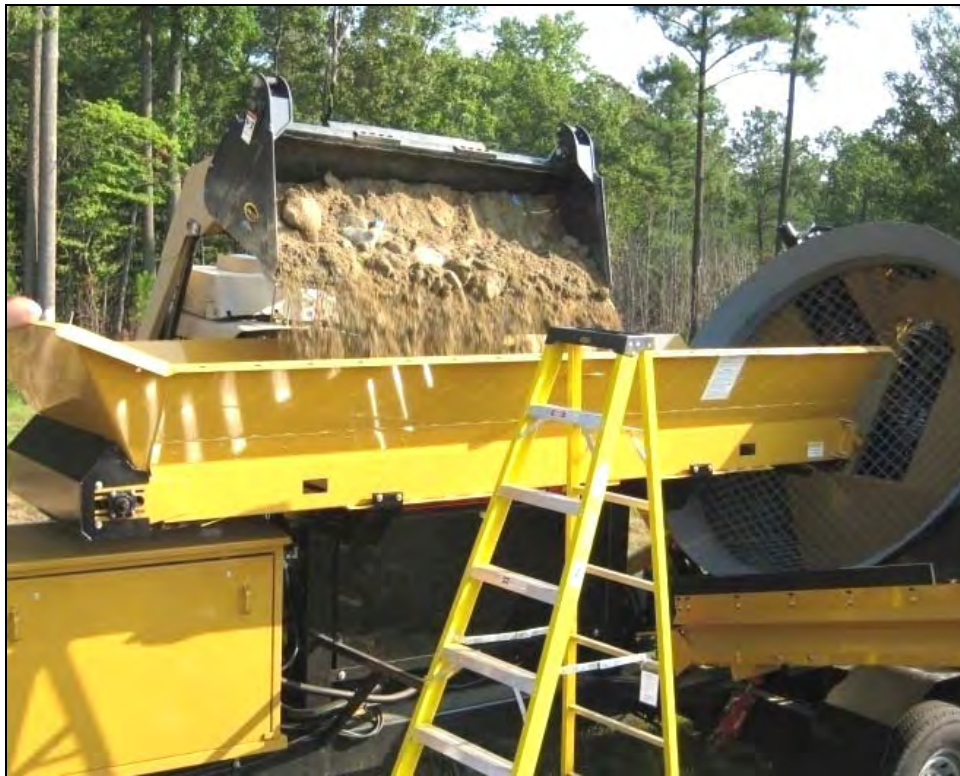
Figure 13: Material Loaded into Sifter's Hopper
