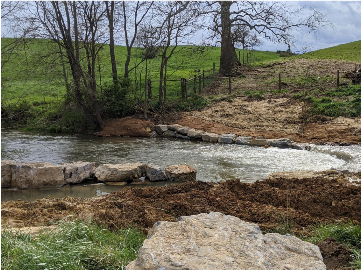
Figure 24. Cross vane implementation side-view Photo by Dylan Cooper, Trout Unlimited
