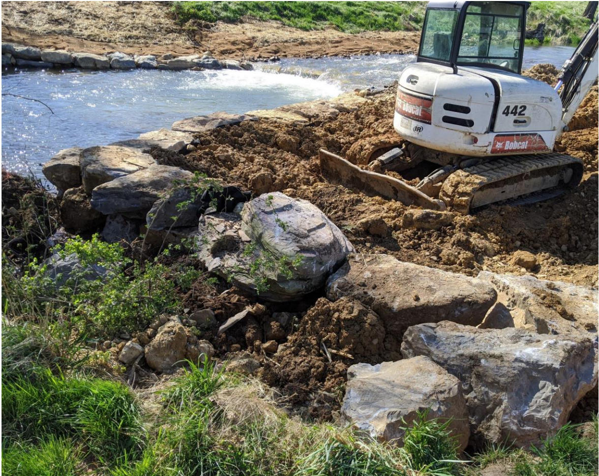
Figure 25. Stabilization of the previously eroded bank Photo by Dylan Cooper, Massanutten Chapter of Trout Unlimited
