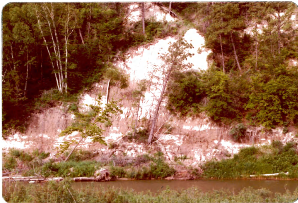
A. Failure of slope.
