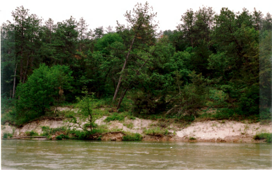
ig. 27. Photograph taken in the summer of 1989, showing the slope failure along the river right of the bridge on the right bank of the river. Sliding and flow is mostly the result of undercutting by water. Although backward tilts of the juniper trees indicate the sliding slumps. The movement is slow but noticeable.
