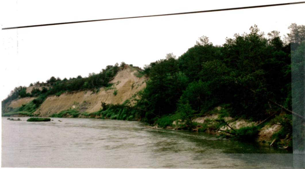
Fig. 26. Slope failure along the Niobrara River. (1) Flow portion with deformed pines (2) Pierre Shale glide blocks (photograph 1989).
