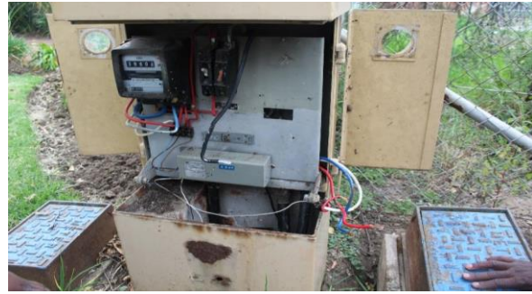
Figure 2.9: Examples of What Meter Tampering Looks Like
