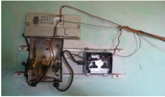
Figure 2.9: Examples of What Meter Tampering Looks Like
