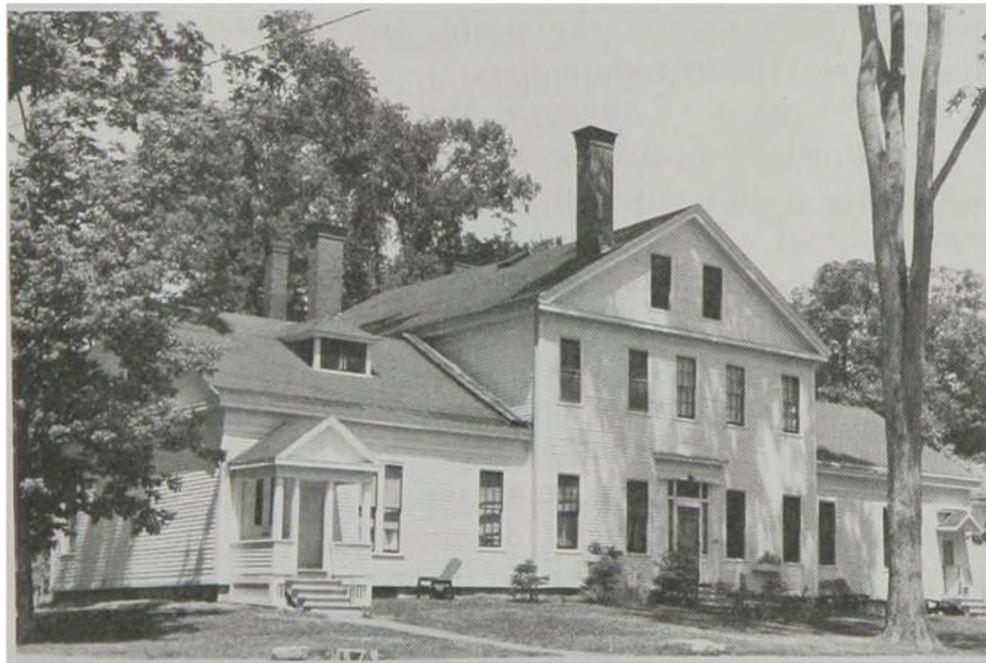
Figure 5 (top): Maine Hall (1833-1834). Figure 6 (bottom): New Commons Hall (1836). Photos by the author.
