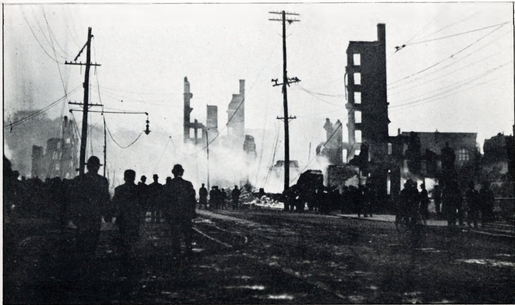
VIEW FROM STATE STREET. RUINS OF MORSE OLIVER BUILDING IN CENTER RUINS OF STEARNS BUILDING ON RIGHT
