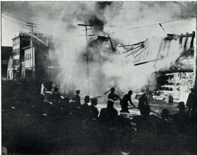
VIEW OF HAY SHED AS THE WALLS FELL
