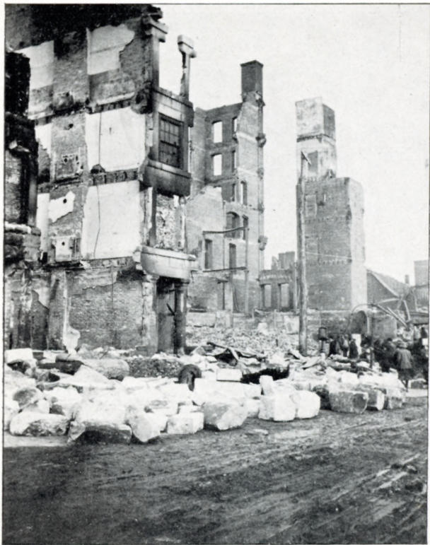
RUINS OF THE MORSE OLIVER BUILDING, SHOWING VAULTS ON THE RIGHT
