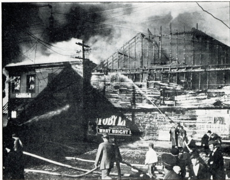
HAY SHED ON BROAD STREET. START OF THE FIRE
