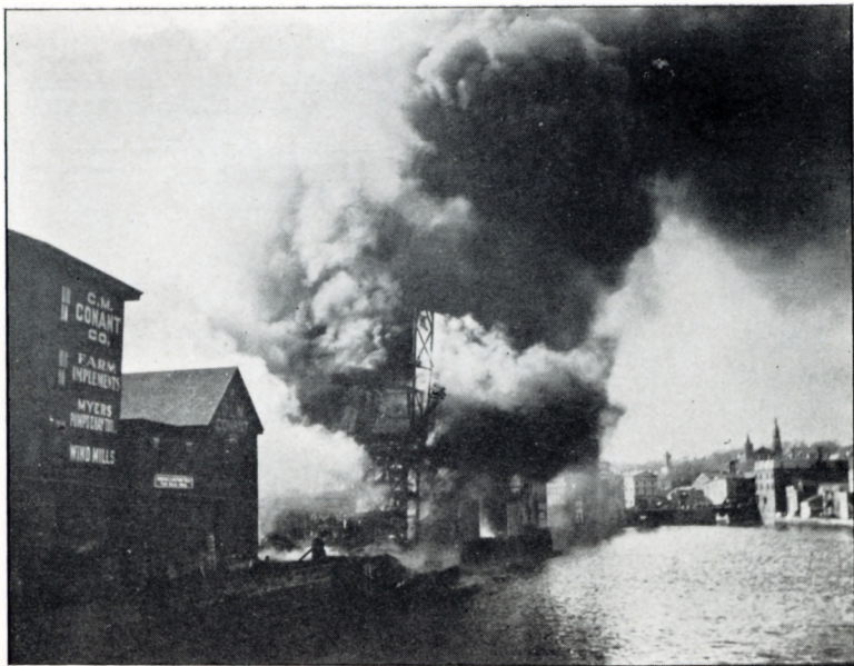
START OF FIRE, VIEW FROM M. C. R. R. BRIDGE
