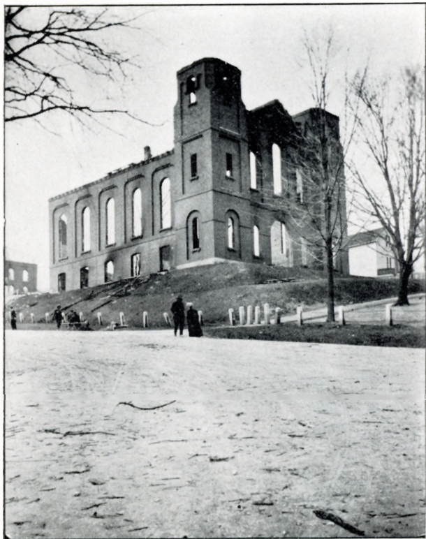
UNIVERSALIST CHURCH, ONE OF THE FIRST PLACES TO CATCH FIRE
