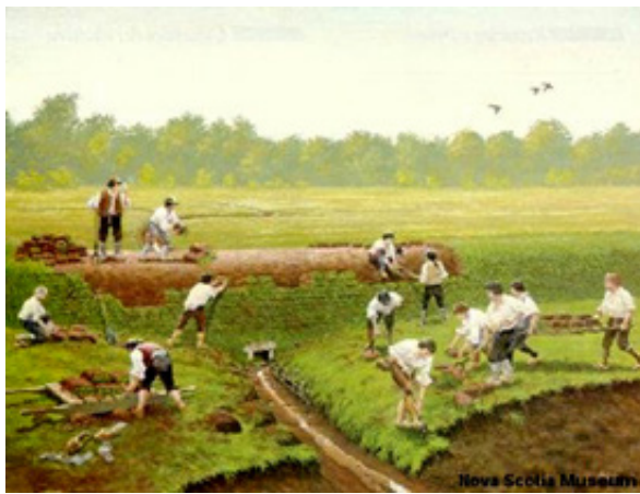
Dike building in Acadia.
