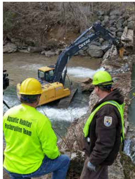
Removal of dam to improve fish passage.
