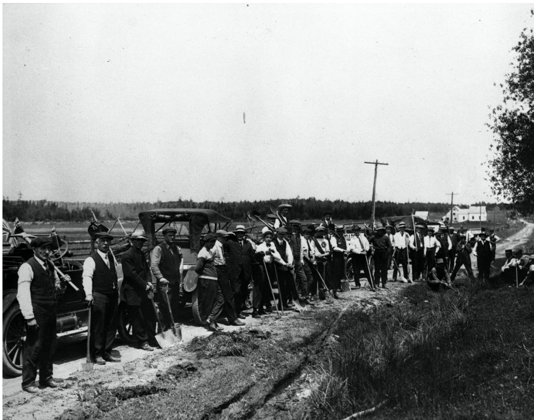
Figure 6- “Good Road Day,” seasonal reconstruction and repair on Shediac Road - June 26, 1913. Courtesy of the Provincial Archives of New Brunswick, Item P75-16.
