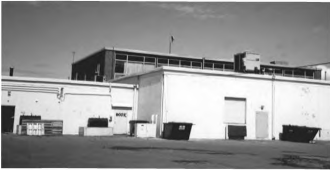
The roof-mounted mechanical equipment (as well as the dumpsters and downspouts) present an unsightly facade in a highly visible location.
