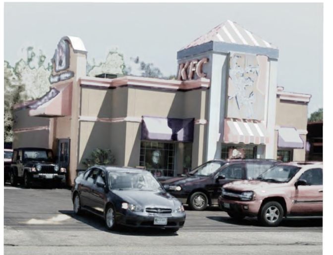
Synthetic stucco (Exterior Insulation and Finish Systems (EIFS))
