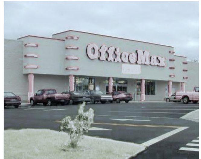
While the front plane of the wall of this building is broken, the offset does not continue to the ground. The projection becomes a billboard and the building is seen as a large box.
