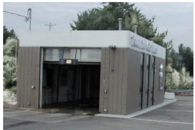
The design of this successful drive-through repeats the same roof pitch, forms, and materials found in the main bank building.
