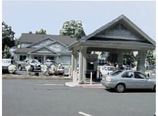
The design of this successful drive-through repeats the same roof pitch, forms, and materials found in the main bank building.
