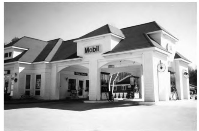
This service station canopy is designed to be an extension of the building. The columns, roofline, dormers, and signage contribute to a sense of continuity in the architecture.
