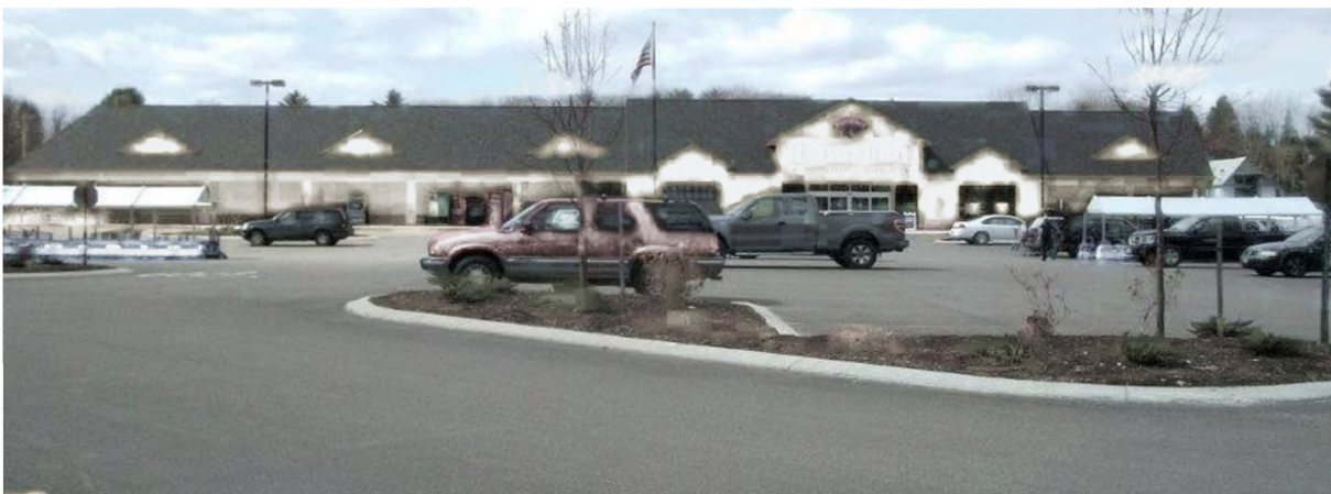
Large retail buildings can be designed to avoid the appearance of a 'big box' through careful massing and detailing.
