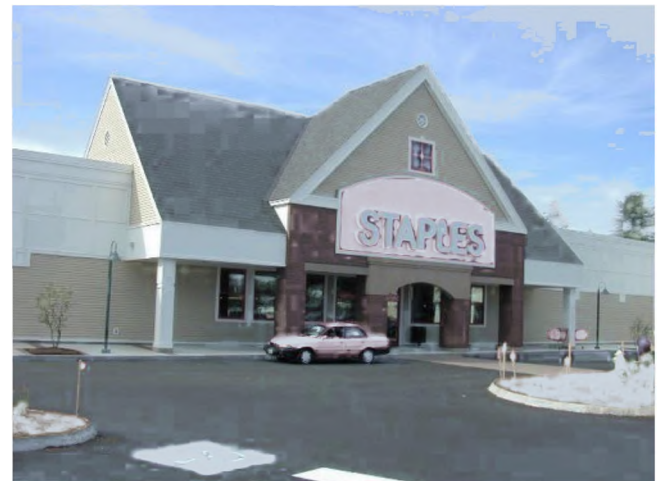
A similar building with a facade composed of New England forms and materials. The overhang provides protection for pedestrians and emphasizes the entranceway. The sign is over scaled (i.e., too large) for the facade.
