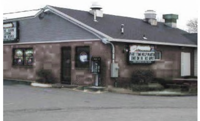
HVAC equipment and service connections are highly visible, adding unnecessary clutter to this small restaurant.
