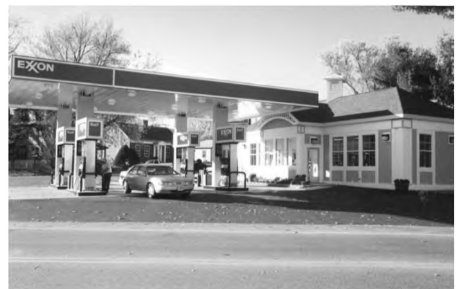
The flat-roofed canopy bears no design relationship to the well-detailed convenience store in terms of form, materials, or architectural style. The store was designed to fit into the residential surroundings.
