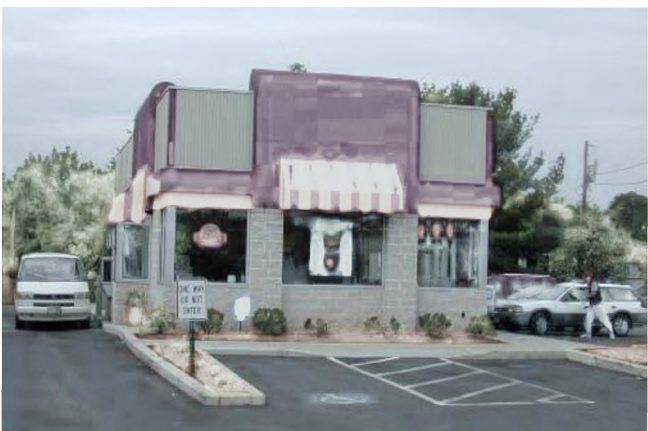
Corrugated plastic panels
