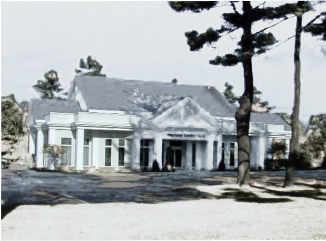
Many elements of New England architecture – pitched roof, gable ends, overhanging roof – are used in this attractive bank building.
