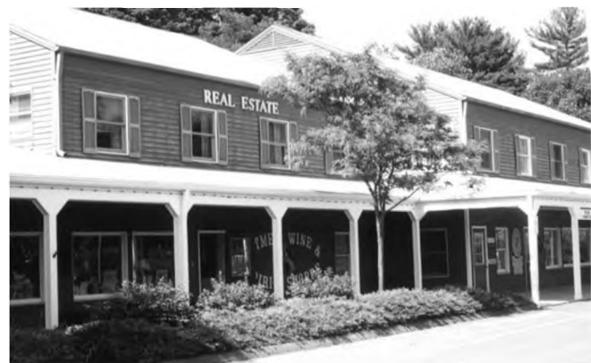
Covered walkways add a shadow line which can reduce the scale
