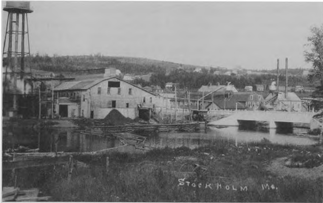
Lumber mills constructed in Stockholm at the turn of the century diversified both the population and the economy, attracting new immigrants and providing opportunities for young Swedes. Author's collection.
