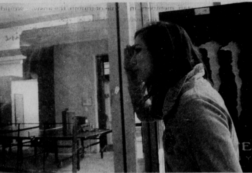
LU Freshman Hallie Virginia Coburn views the new construction. Photo By: Baylee Holman
