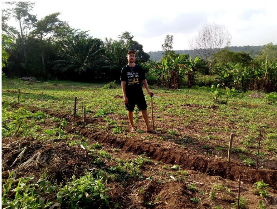
Figure 7: Newly constructed earthen berms installed by author with a farming hoe at the top border of each plot. (Photograph taken by the author)
