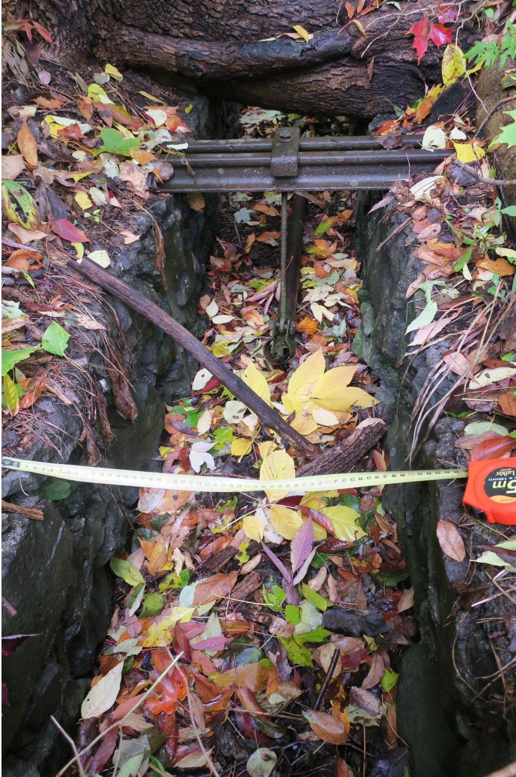
Figure 6.31: Photo of Feature 263 facing east, showing a rail holding brackets that hold an iron pipe.
