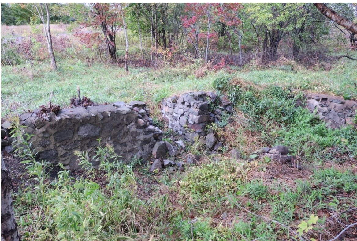
Figure 6.48: Photo of Feature 30 facing south, showing an entrance to the structure.
