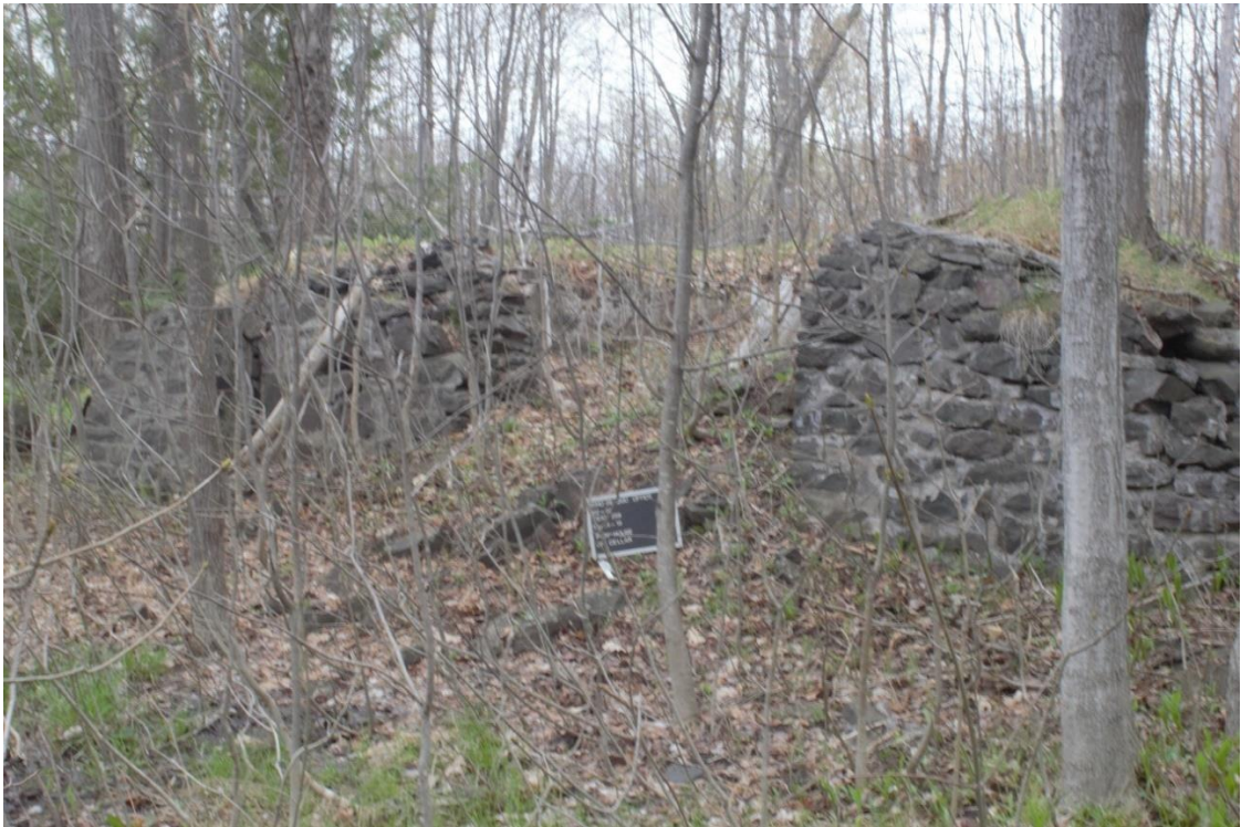
Figure 6.16: Photo of the stone walls of F259 facing northwest.
