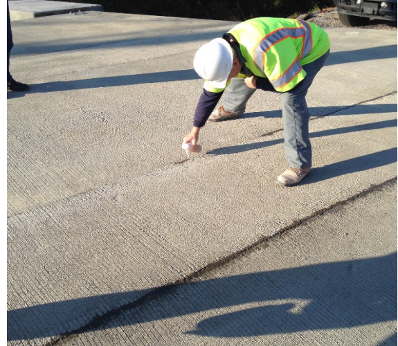
Figure 19 Applying methyl-methacrylate crack sealer to cold joint at tie pour
