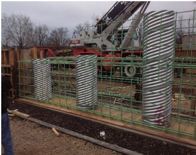
Figure 12 Forming abutment caps for casting in laydown yard
