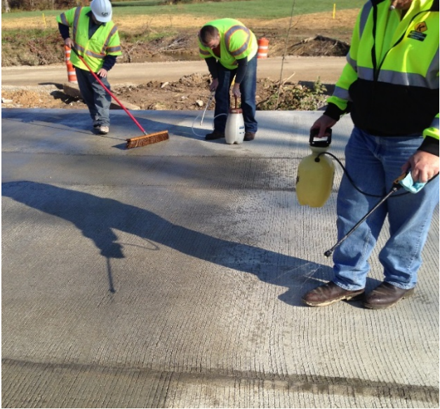
Figure 22 Application of penetrating deck sealer
