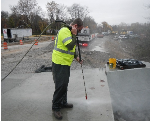
Figure 18 Cleaning bridge deck with 5,000 psi wash
