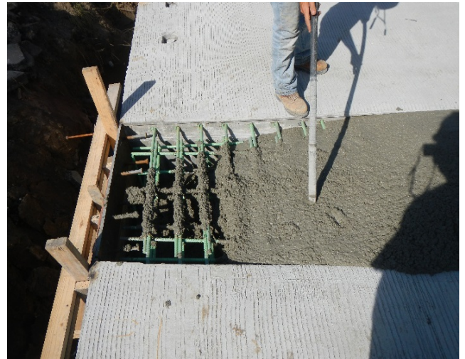
Figure 17 Class M concrete used to tie precast deck panels together
