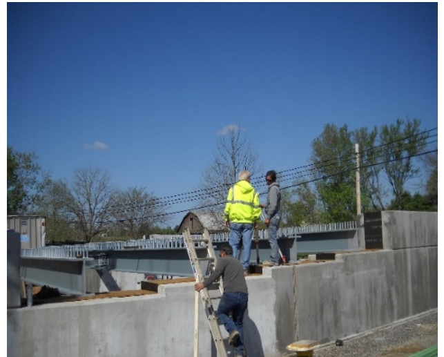
Figure 13 Preassembling painted beams on precast abutments
