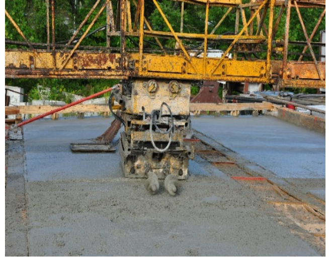
Figure 15 Casting deck panels at laydown yard
