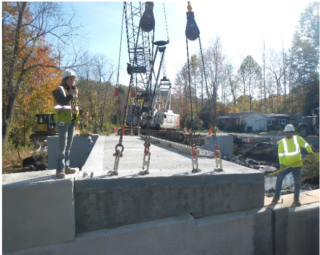
Figure 16 Precast deck panel placed on precast abutment cap
