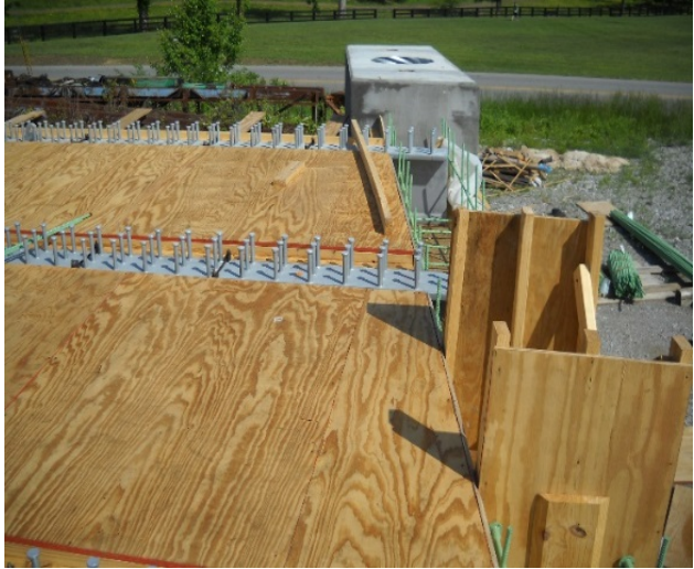
Figure 14 Formwork to cast deck panels at laydown yard
