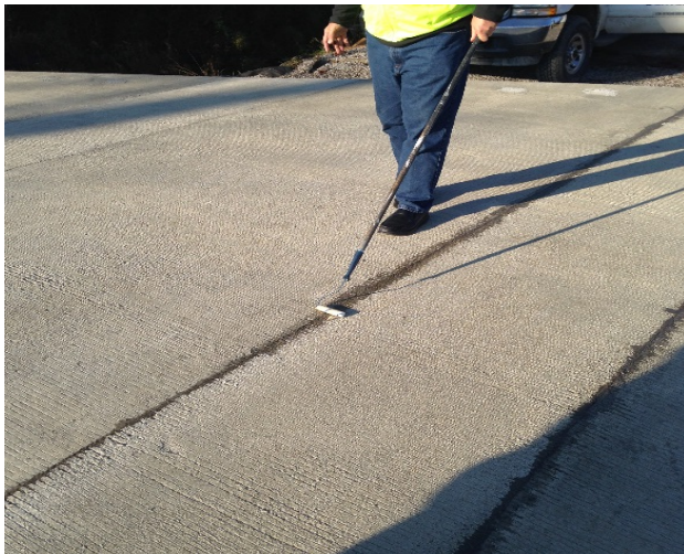
Figure 20 Spreading and smoothing crack sealer with a roller
