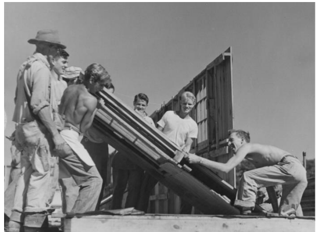
Figure 5.4: Student veterans construct housing in Shawneetown (1946)
