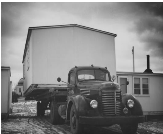
Figure 5.5: Two men haul temporary housing buildings for Cooperstown (1946)
