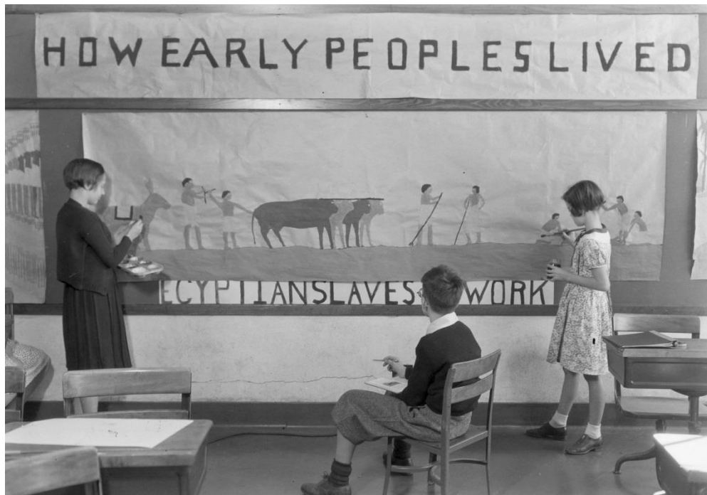
Figure 4.46: UK Teacher Training School: Students learn about the development of civilization by depicting Egyptian slaves at work (University of Kentucky Archive)
