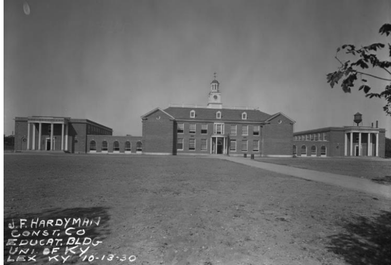
Figure 4.15: The front of UK Teacher's Training School on October 13, 1930.
