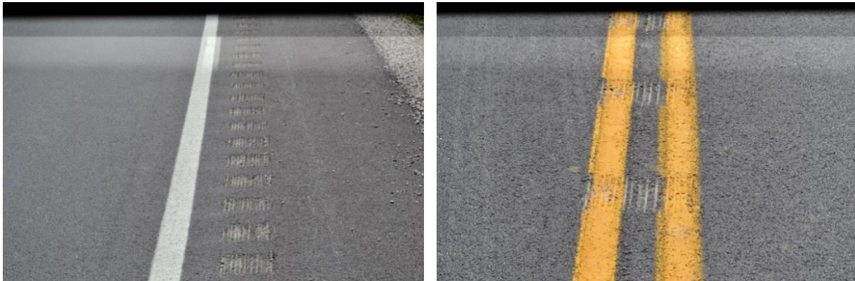
Figure 5.15 US-27 Rough Cut Centerline and Shoulder Rumble Strips
