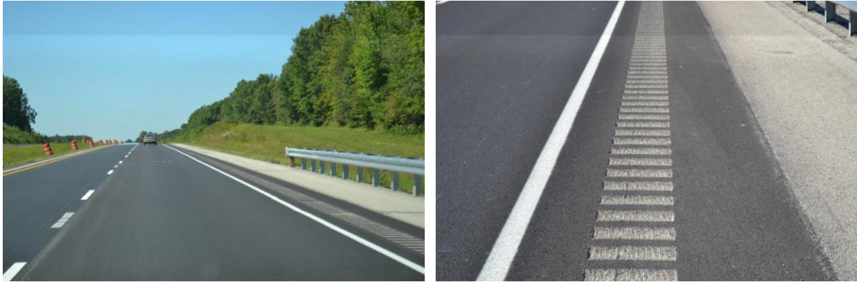
Figure 5.3 Kentucky Shoulder Rumble Without Bicycle Gap
