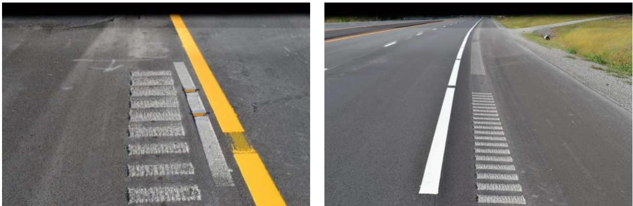
Figure 5.2 Kentucky Shoulder Rumble with Bicycle Gaps
