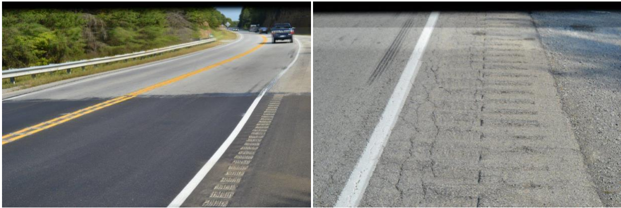
Figure 5.20 KY-245 New vs. Old Shoulder Rumble Strips
