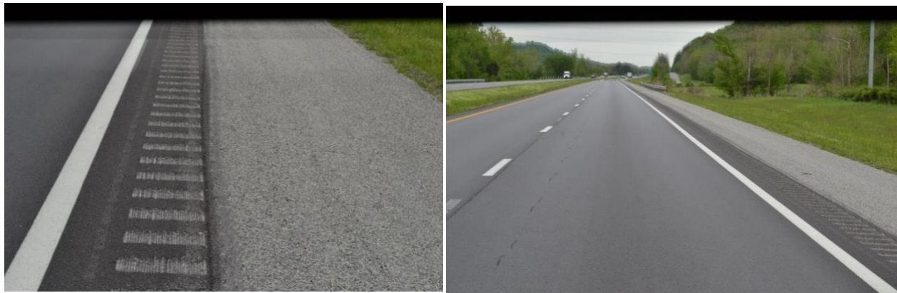
Figure 5.18 Bluegrass Parkway Shoulder Rumble Strip
