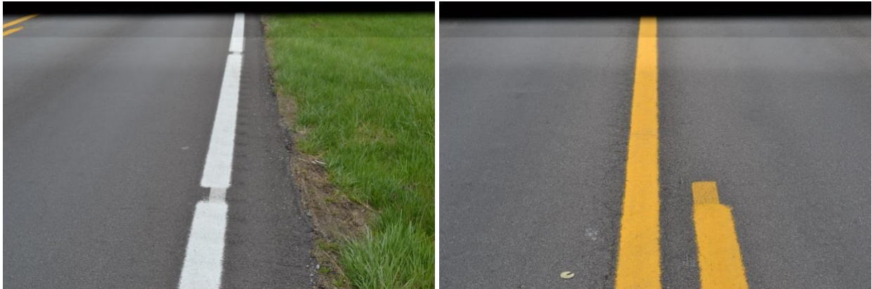
Figure 5.13 US-60 Thin Overlay on Existing Edgeline Rumble Strip
