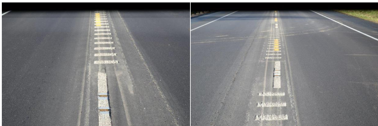
Figure 5.9 Mountain Parkway Centerline Rumble Strip and Recessed Markers
