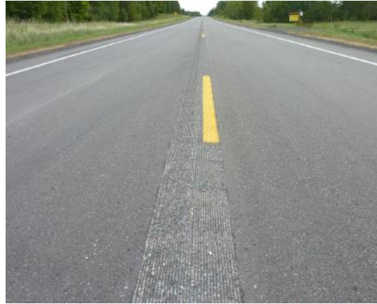
Figure 2.2 Minnesota DOT, Design 1 Sinusoidal Rumble Strips
