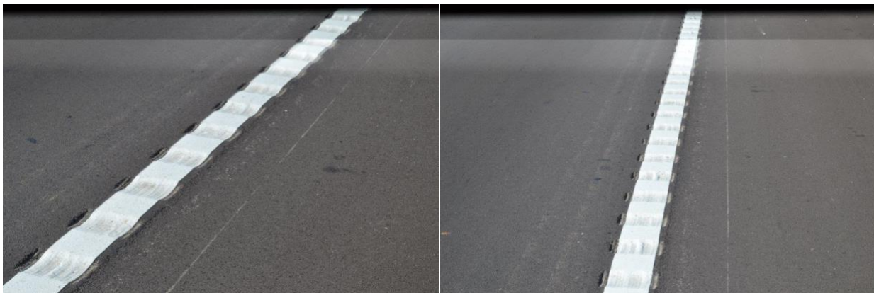
Figure 5.11 New Circle Thermoplastic Edgeline Rumble Strip
