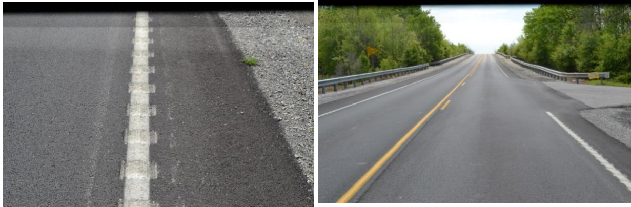
Figure 5.17 US-62 Edgeline Rumble Strip on a Narrow Shoulder
