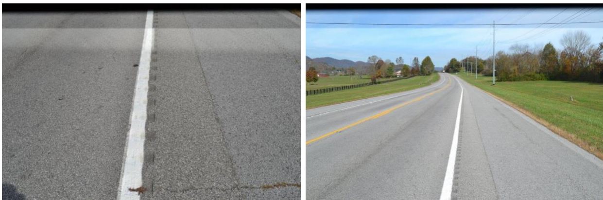
Figure 5.22 RT-63 Shoulder Rumble Strip Moved to Edgeline
