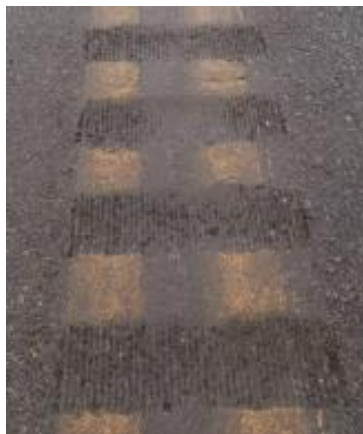
Figure 2.3 Minnesota DOT, Conventional Rumble Strips
