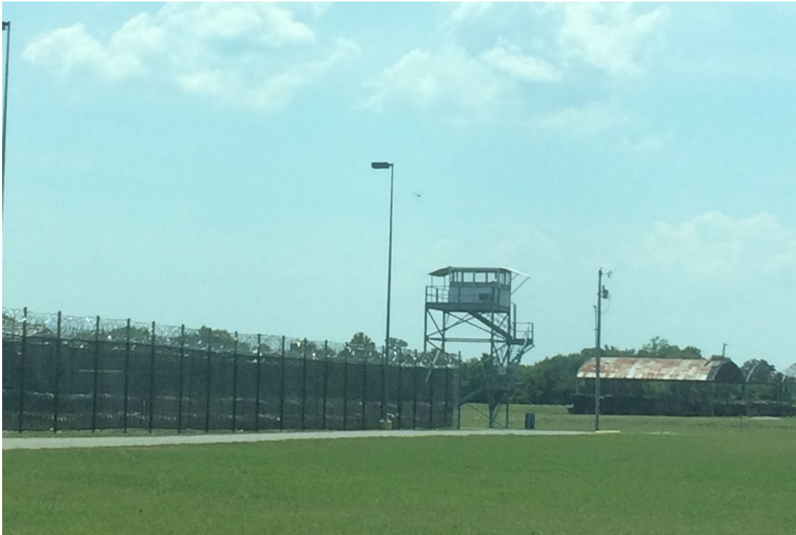
Figure 6: Guard tower at the former youth prison and the remnants of an outbuilding from Chicago Mill and Lumber.
