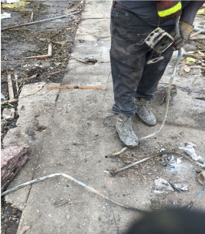
Figure 13: Pulling copper wire from electrical conduit.
