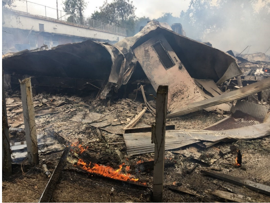
Figure 11: Razed trailer featuring a metal door and tin roof.
