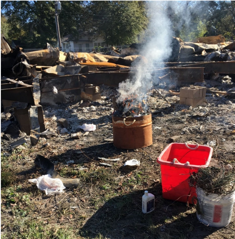
Figure 16: Copper wire being burned to remove casings.
