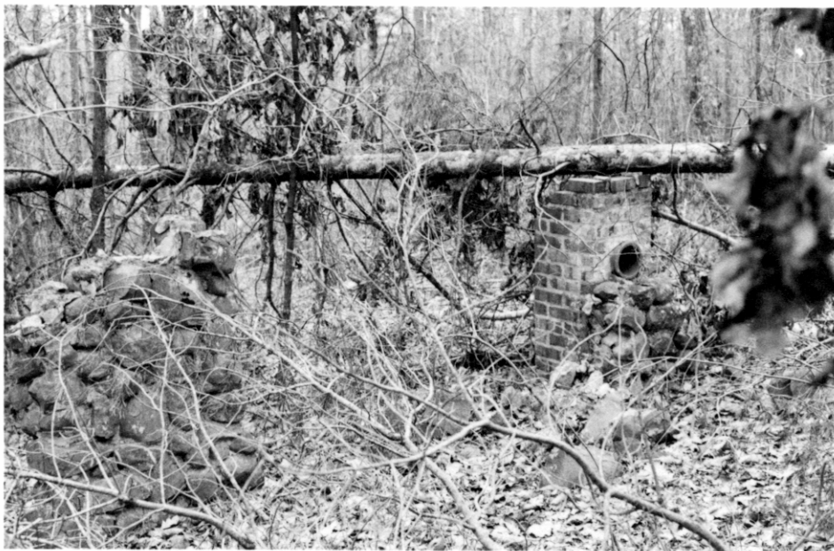
Figure 8. View of Foundation Ruins at Rd835
