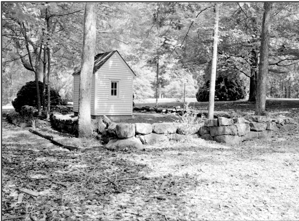
Figure 8. Stone foundation looking southeast.
