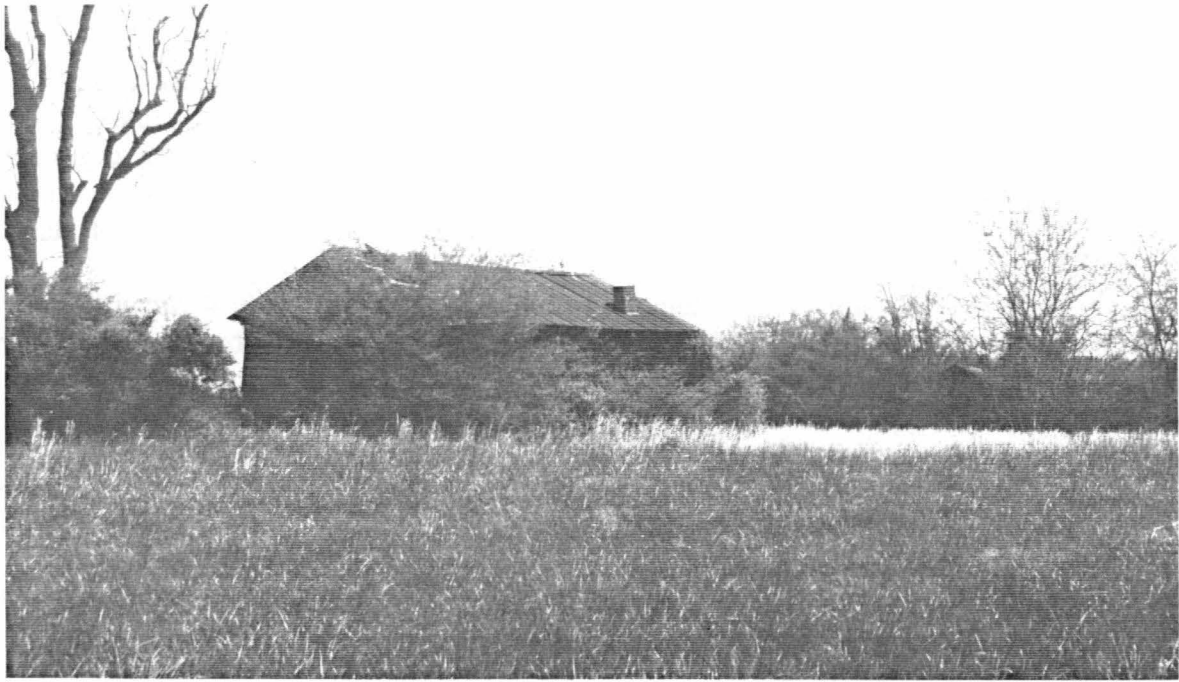
Figure 8. Close-up view of Structure 1 at site 31Mk632 (view to east).
