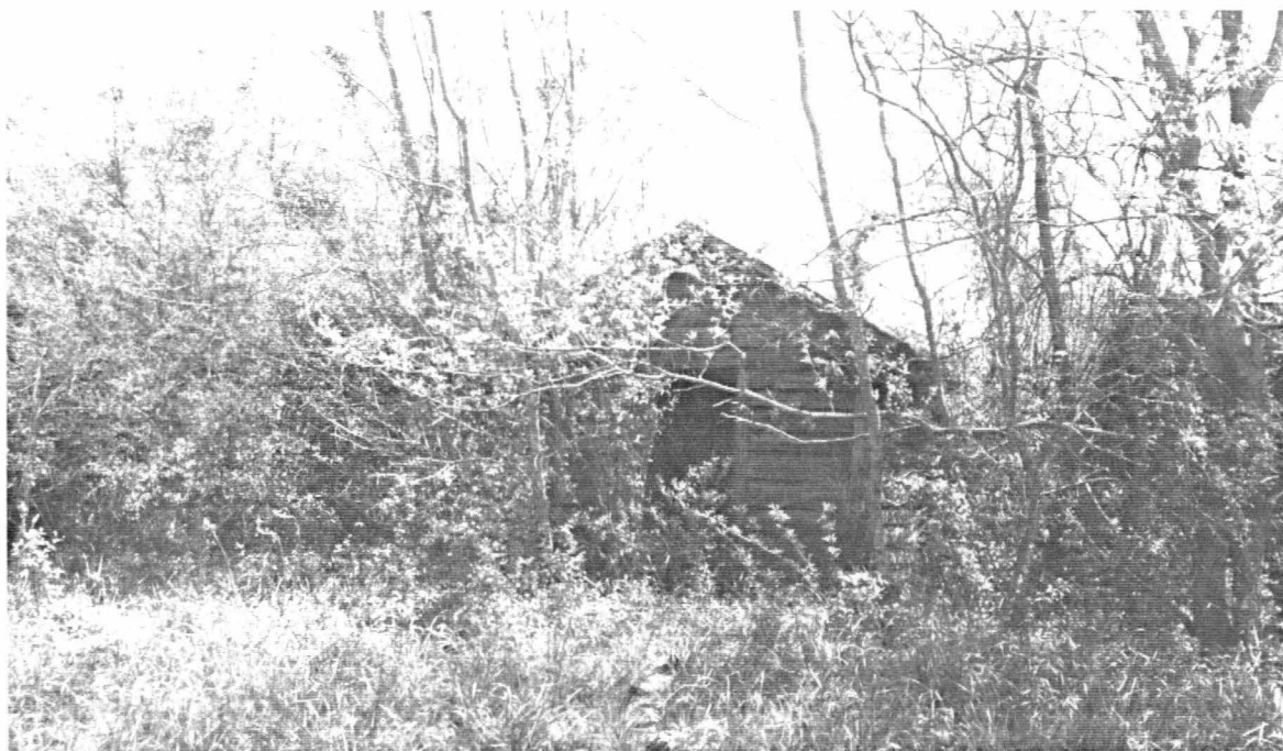
Figure 10. Close-up front view of Structure 3 at site 31Mk632 (view to southeast).
