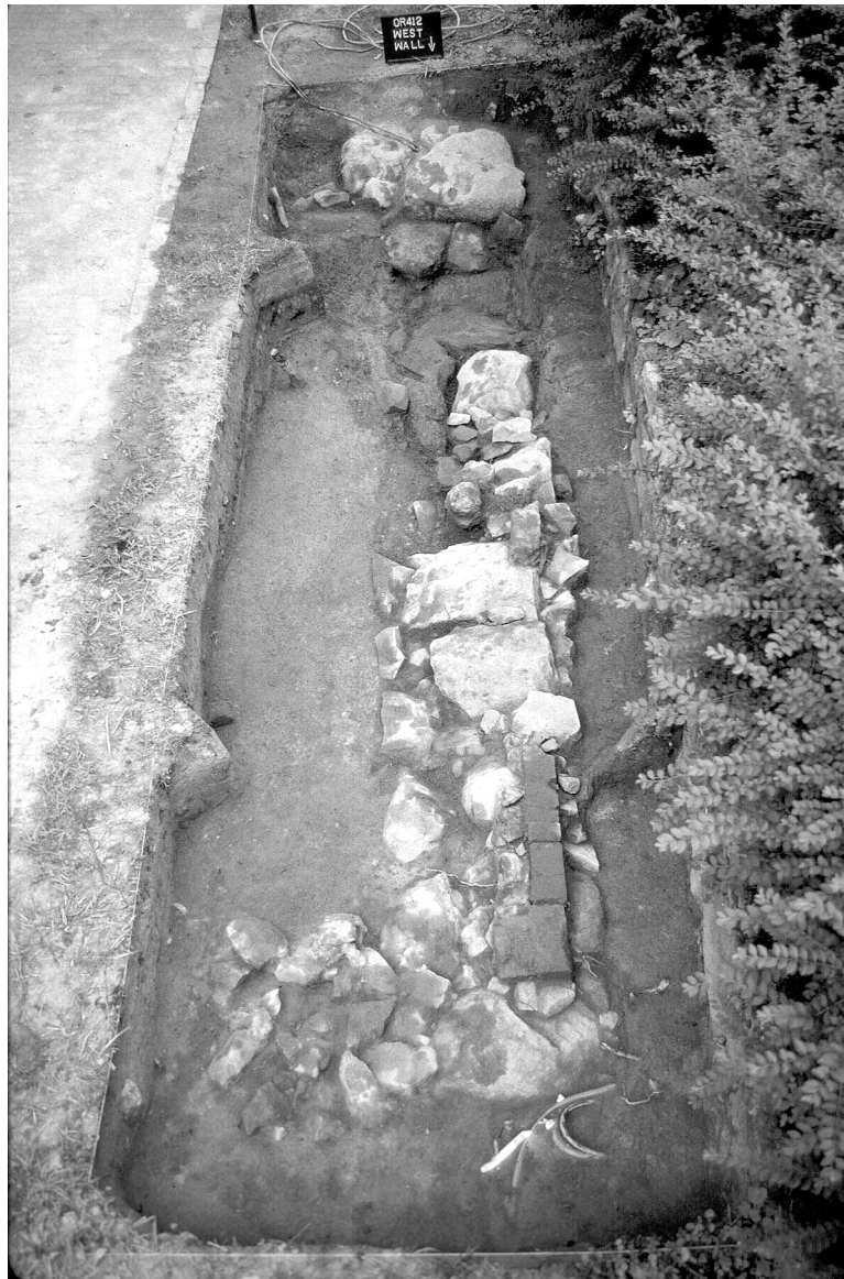
Figure 29. West wall foundation of Structure 2 showing intact course of bricks in foreground (view to south).
