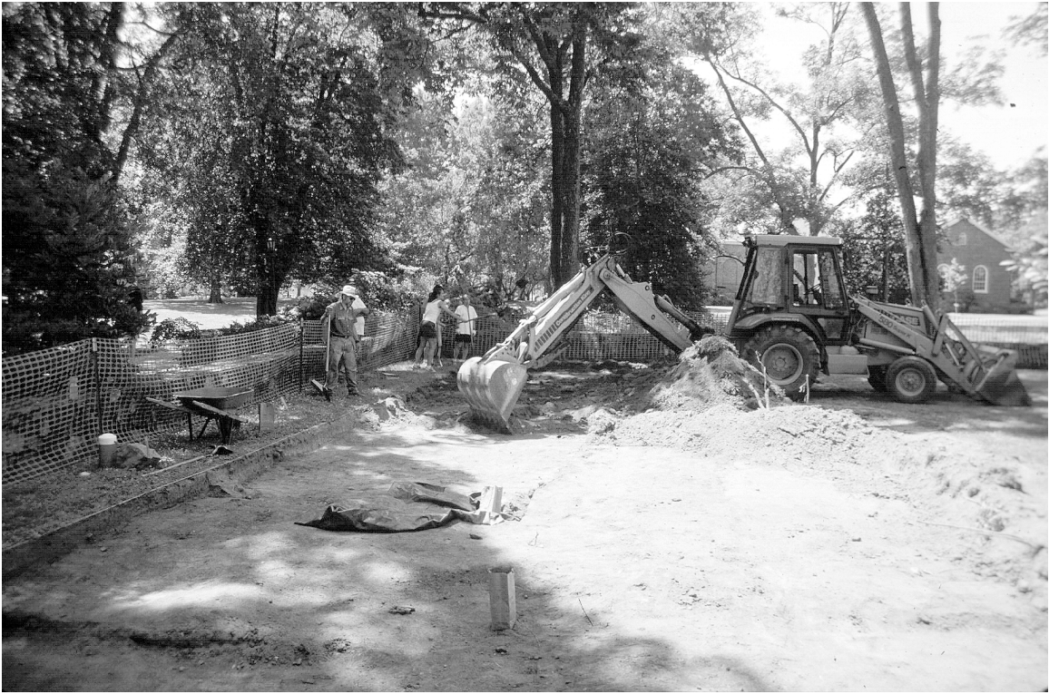
Figure 20. Removing topsoil from the Pettigrew site with a backhoe (view to south).
