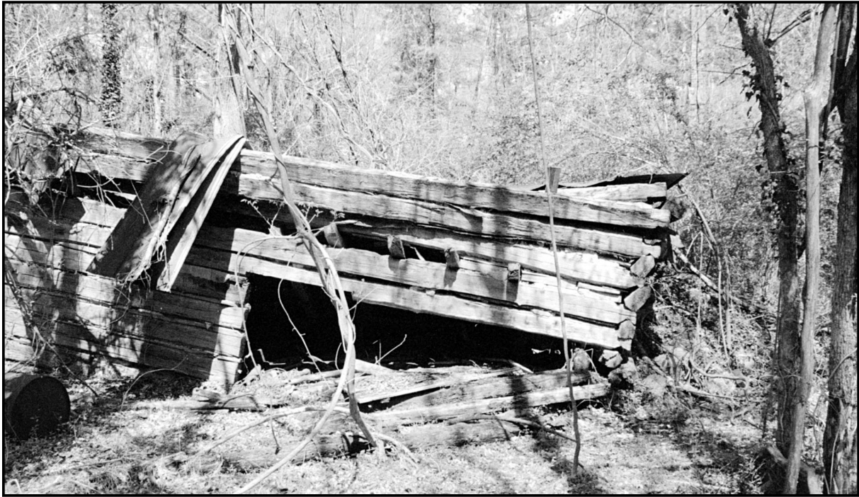
Figure 5.16. Site OR450, Structure 1.
