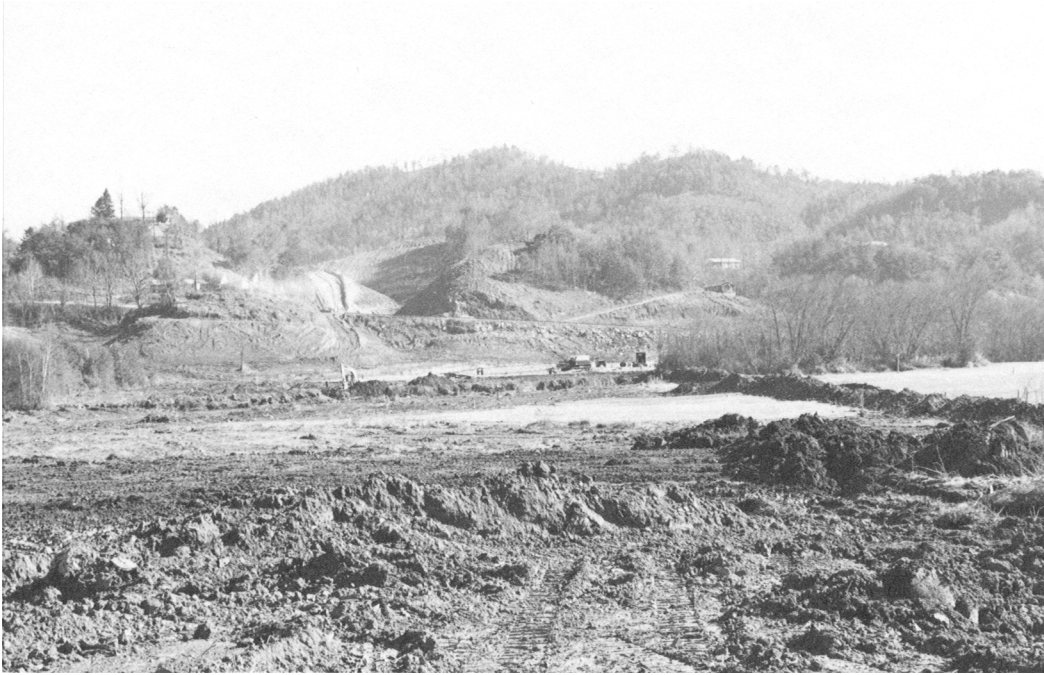
Plate I Road Construction Through Wood's Bottoms Near Andrews
