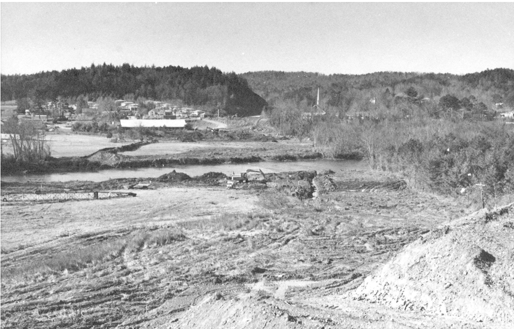
Plate II Construction on the Hiawasse River Bridge Just Outside Murphy
