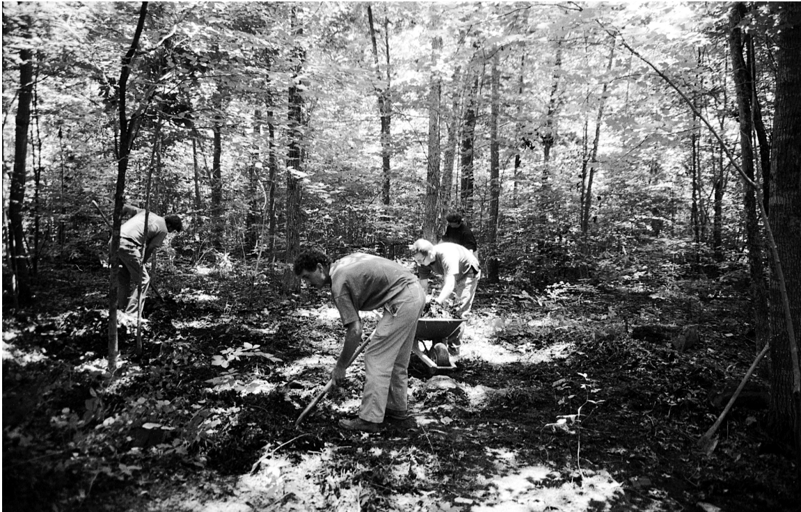
Figure 1. Clearing foundation remains at the Davis cabin site. [substituted for original]
