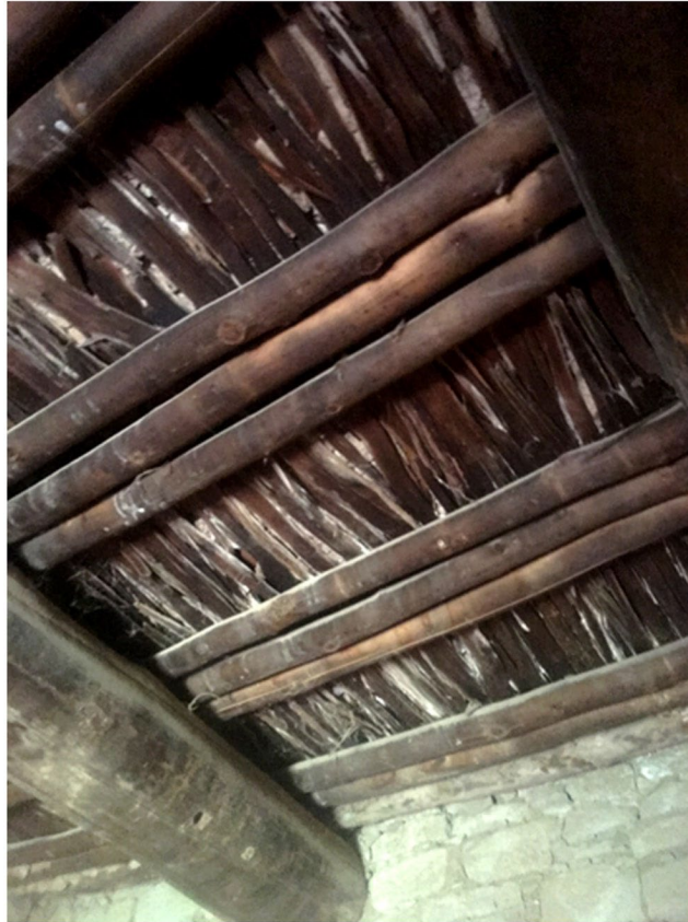
Fig. 8. Detail of one of Aztec Ruins' room ceiling showing the complex organization of the wood that probably resulted in the protection of the coprolites and hampered the parasite egg degradation in Room 225. Photo: Morgana Camacho.
