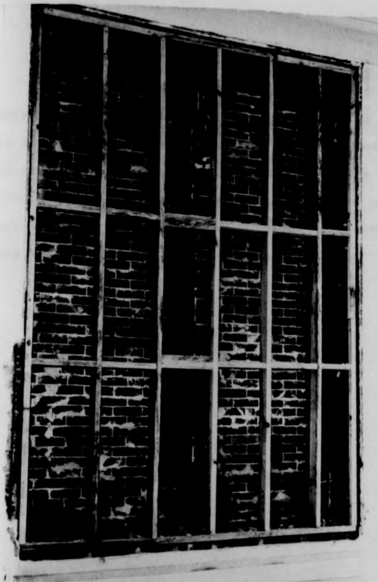
Figure 24. South Central Bedroom on East Wall with Double Window Closed Off
