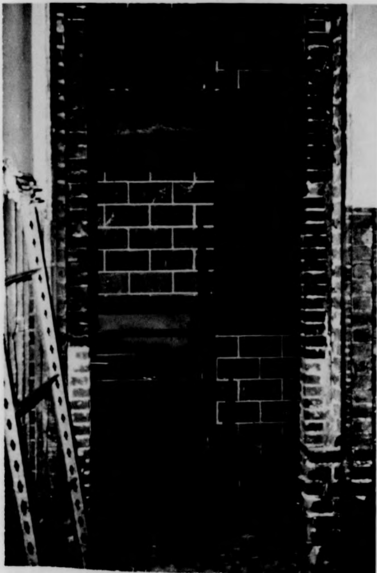
Figure 20. Interior Entrance on the Second Floor to the Stair Tower/Fire Escape
