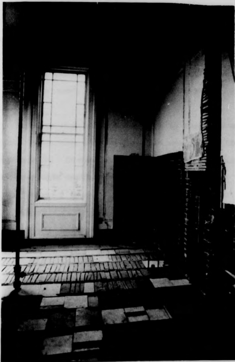
Figure 46. Initial Layer of Flooring
