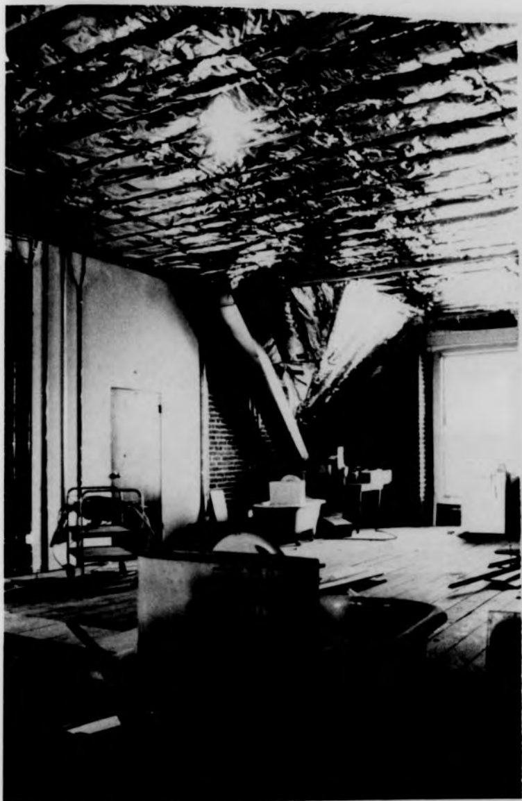
Figure 44. Insulation of the Third Floor in an Unfinished Area
