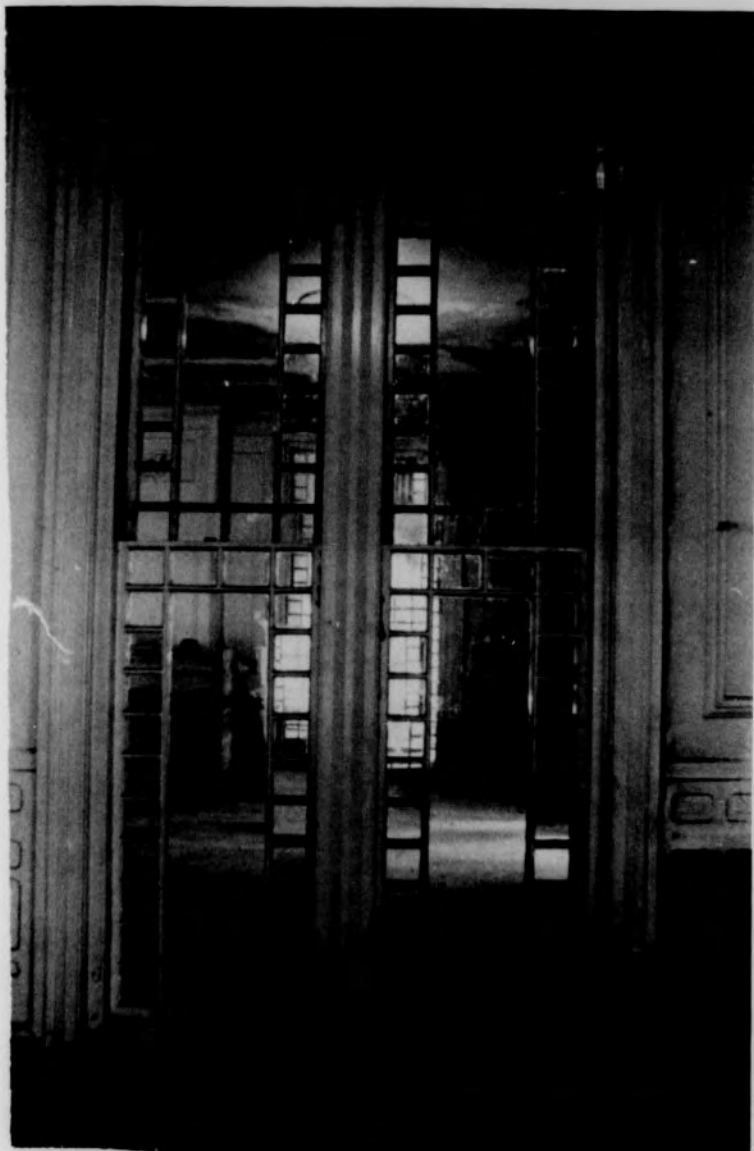
Figure 22. Ballroom Double Window on East Wall with Silver Mirror Replacement
