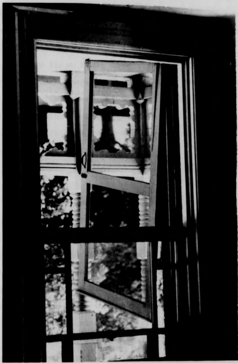
Figure 12. Second Floor Balcony Window and Hinged Screen
