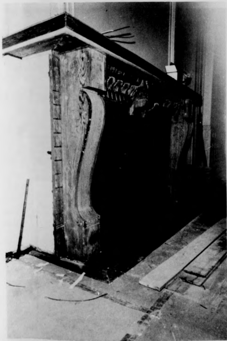
Figure 42. Fireplace Mantel Stripped of Paint and Reset in Wall
