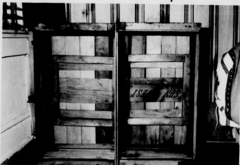
Figure 9. Seat platform inverted showing reinforcement.
