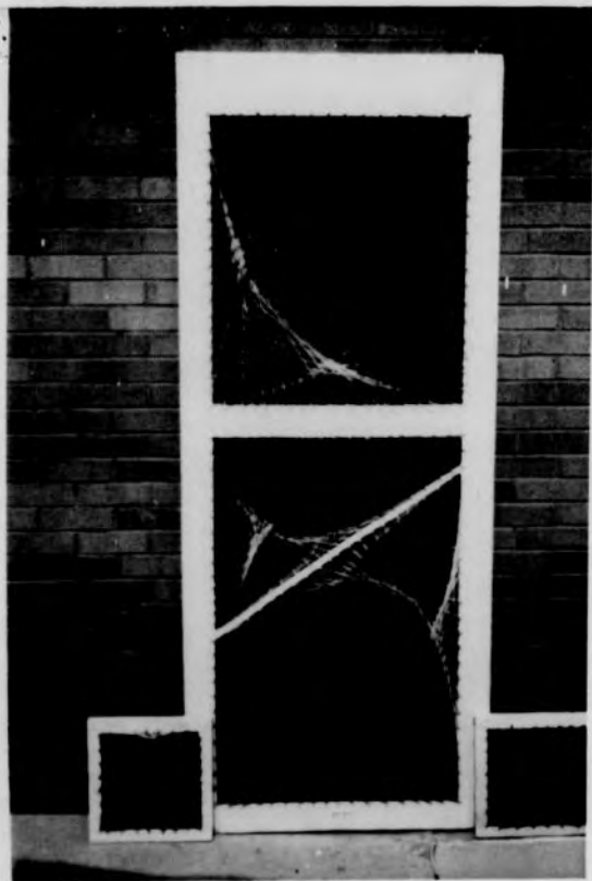
Figure 47. Screens made from melon crates and a screen door that could be used to frame a window seat.
