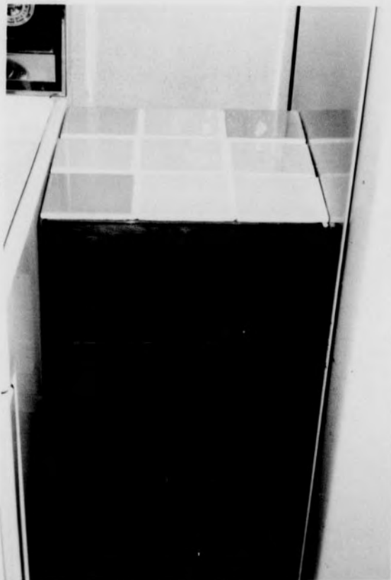
Figure 24. Counter with a tiled surface made from two crates nailed together.
