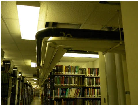
Figure 1: The ceiling of the library basement pre-construction
