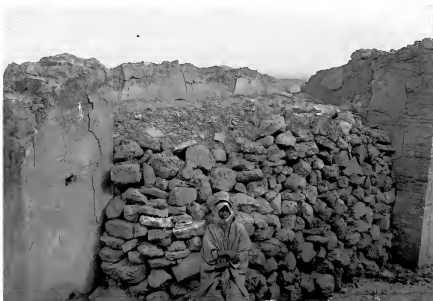
Figure 2.3: Rocks and fill applied against wall paintings to protect them until they were removed, Temple of the Palmyrene Gods, 1930–31. Yale University Art Gallery, Dura-Europos Collection
