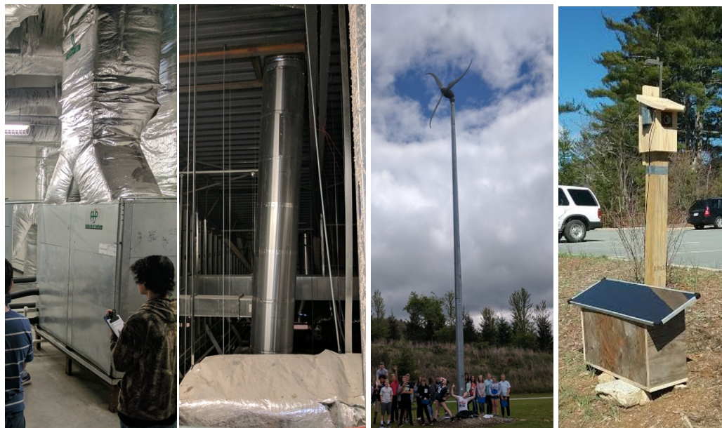
Figure 17. Renewable energy school tour. From left to right: geothermal heat pump system, solar tubes, wind turbine, solar powered camera and photo transmitter on bird house.
