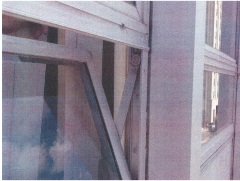
Figure 61. Original Operational Windows on the Motor Lodge Bedrooms. (Hills, 2016)
