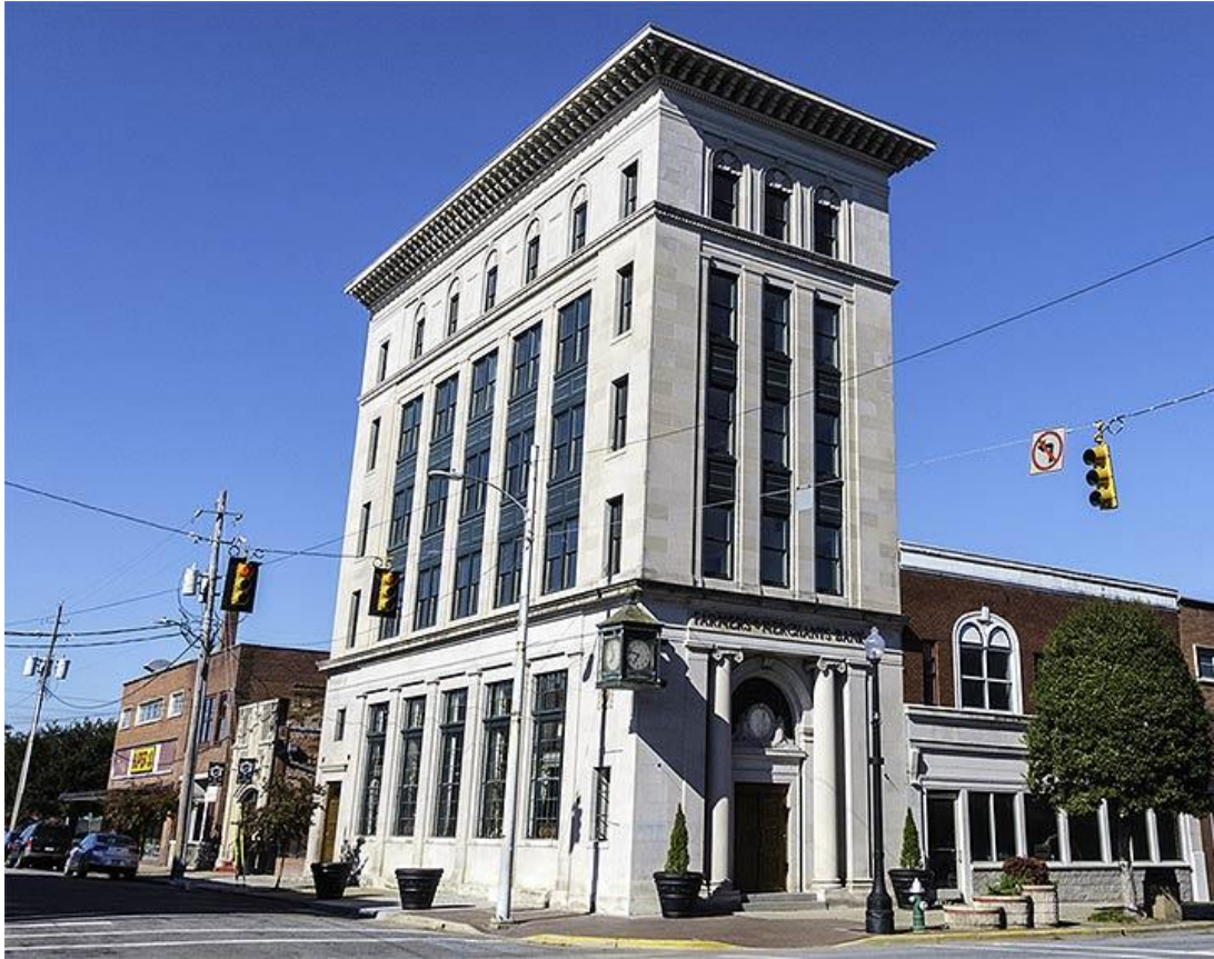
Figure 9. The O'Neil Hotel Façade. (The O'Neil Boutique Hotel, 2015)
