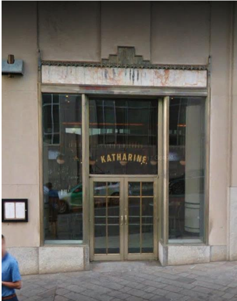
Figure 32. Current Restaurant Entrance. (Heritage Construction Group, 2016).
