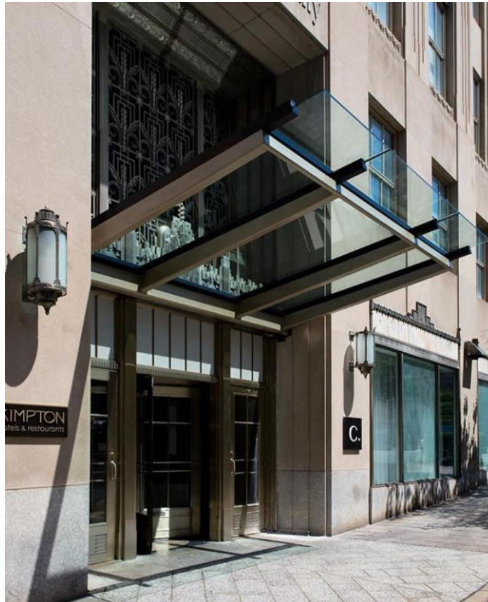
Figure 31. West Entrance with Canopy Addition. (Expedia, n.d.).
