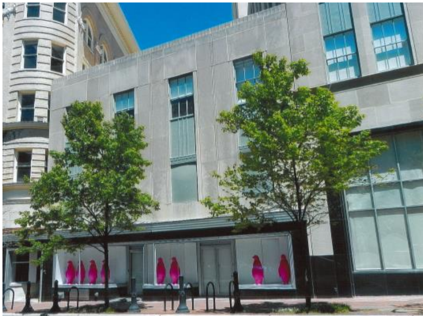
Figure 42. Cleaned Façade of the Hill Building. (Greenberg, 2013a).
