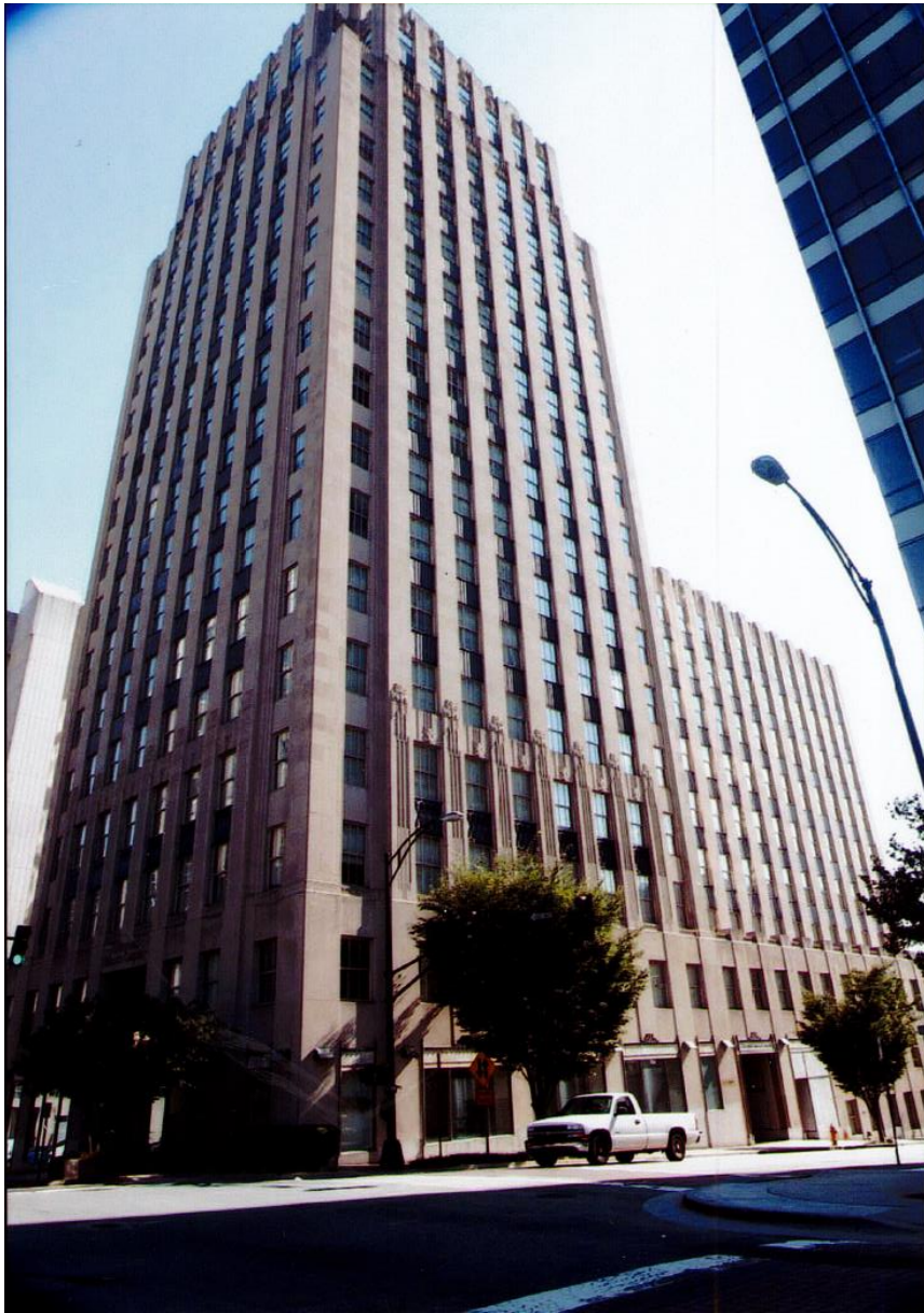
Figure 28. Before Image of the West (Main Street) Façade. (Heritage Construction Group, 2016).
