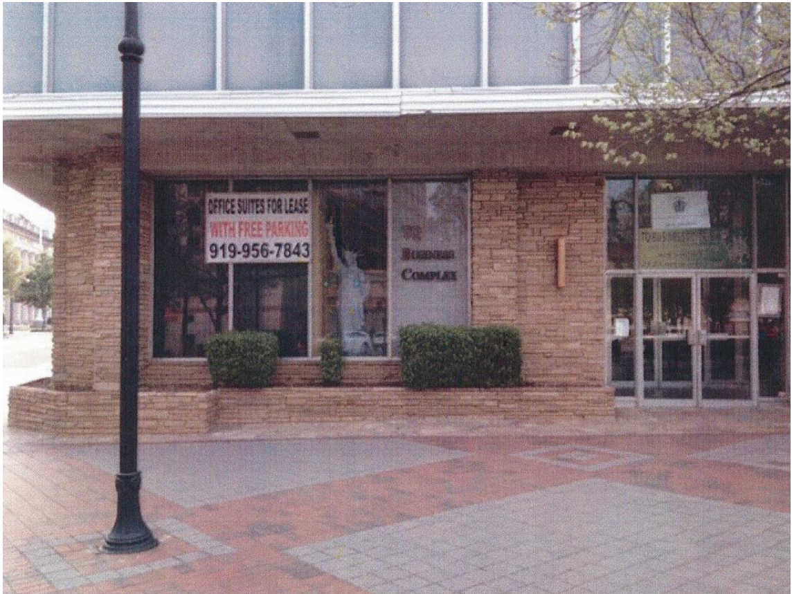
Figure 56. Façade of the Jack Tar Motor Lodge Before the Adaptation. (Hills, 2016).
