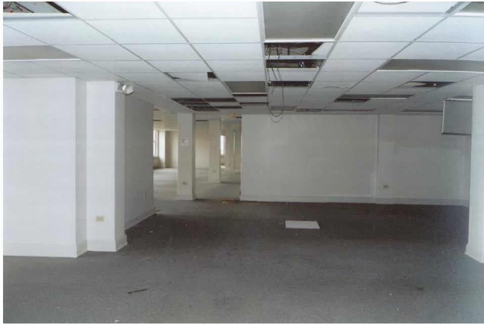
Figure 46. Former Second-Floor Office Space. (Greenberg, 2013a).
