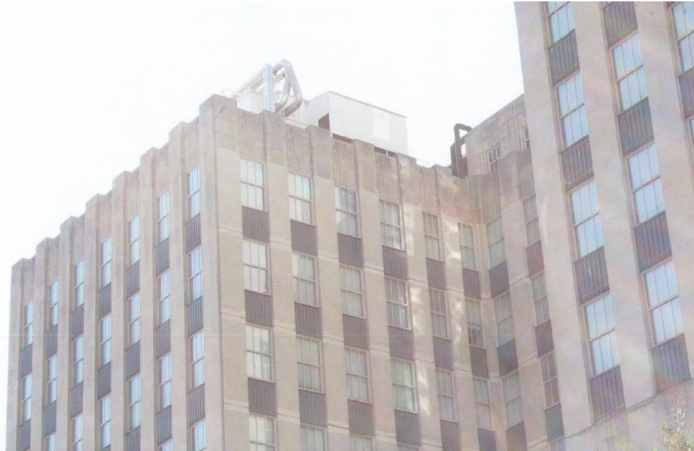
Figure 34. Upper Floor Windows Before the Adaptation. (Heritage Construction Group, 2016).
