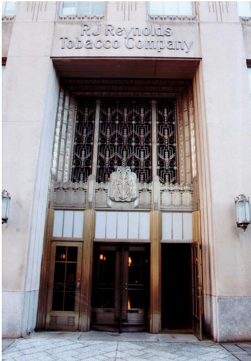
Figure 30. Before Image of the West Entrance without the Canopy. (Heritage Construction Group, 2016).
