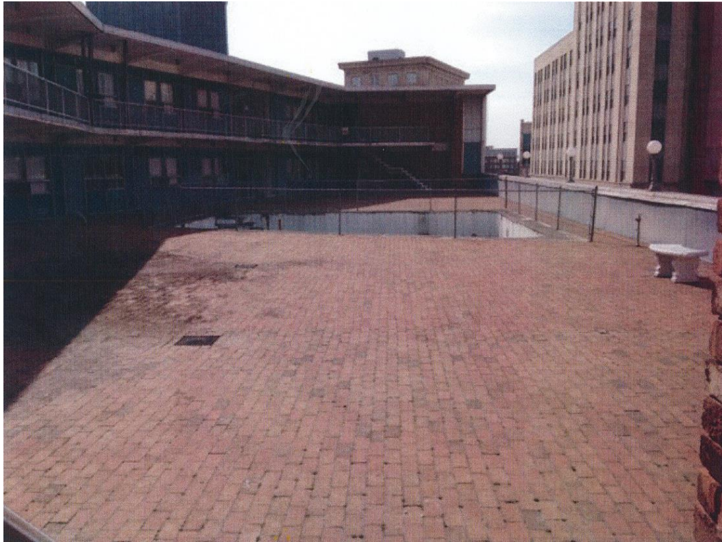
Figure 67. Paver on the Roof Deck Prior to Rehabilitation. (Hills, 2016).
