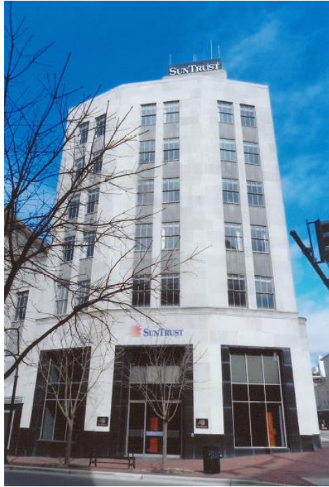
Figure 41. Black Granite on Storefront Façade. Original Condition (Greenberg, 2013a).
