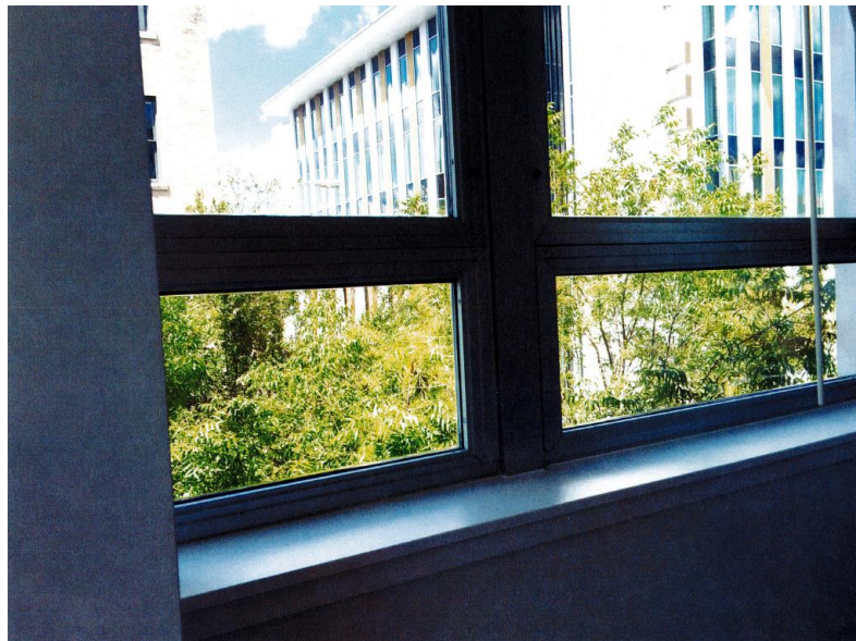
Figure 62. The New Windows. (Hills, 2016).
