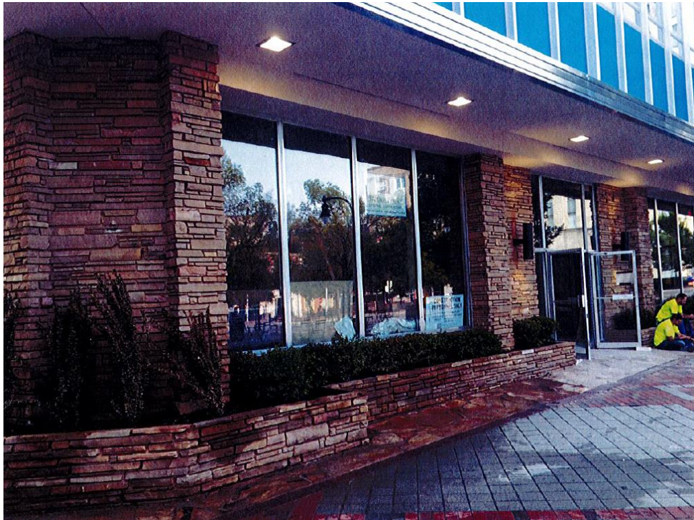
Figure 57. Part of the West Façade Tan-colored Stone After the Restoration. (Hills, 2016)
