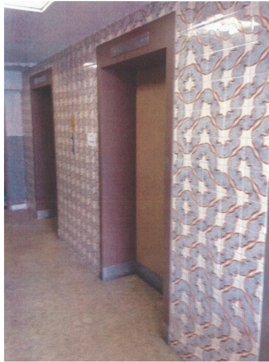
Figure 65. Elevator Lobby with Original Tile. (Hills, 2016)
