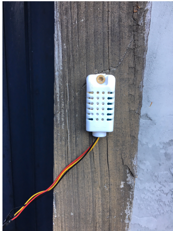
Figure 4. The DHT22 temperature and humidity sensor, shown mounted on a wooden post outside of the control room.
